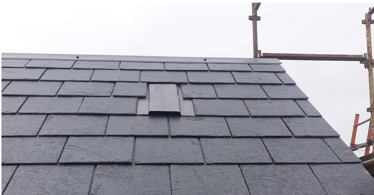
Plate 3: Bat slate (one of two inserted into roof space).
