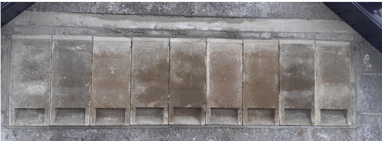
Series of Bat Tubes inserted into the external wall of Oldstreet Substation Bat House, Co. Galway (pre-plaster).
