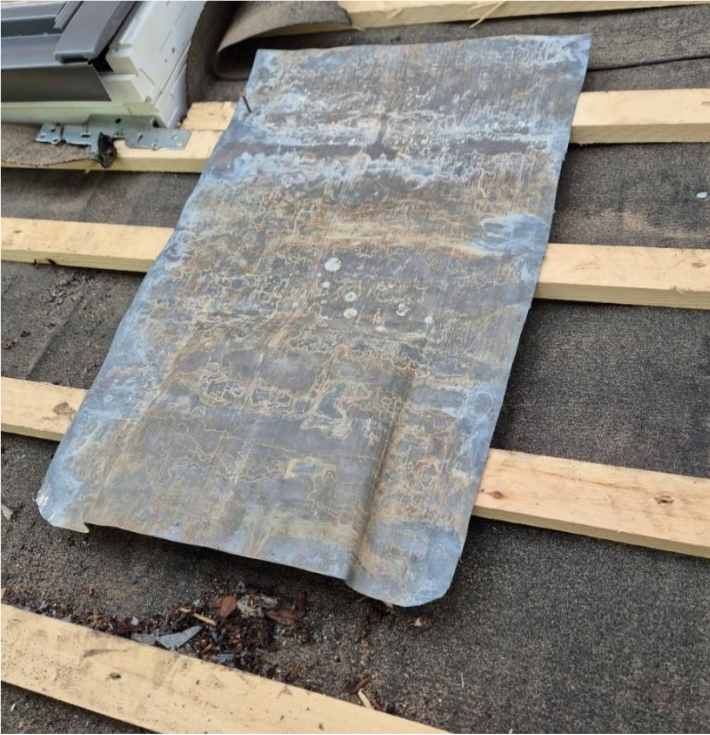
Construction of bat slates for inspection by bat specialist at Coole Park Visitor Centre, Gort, Co. Galway.
