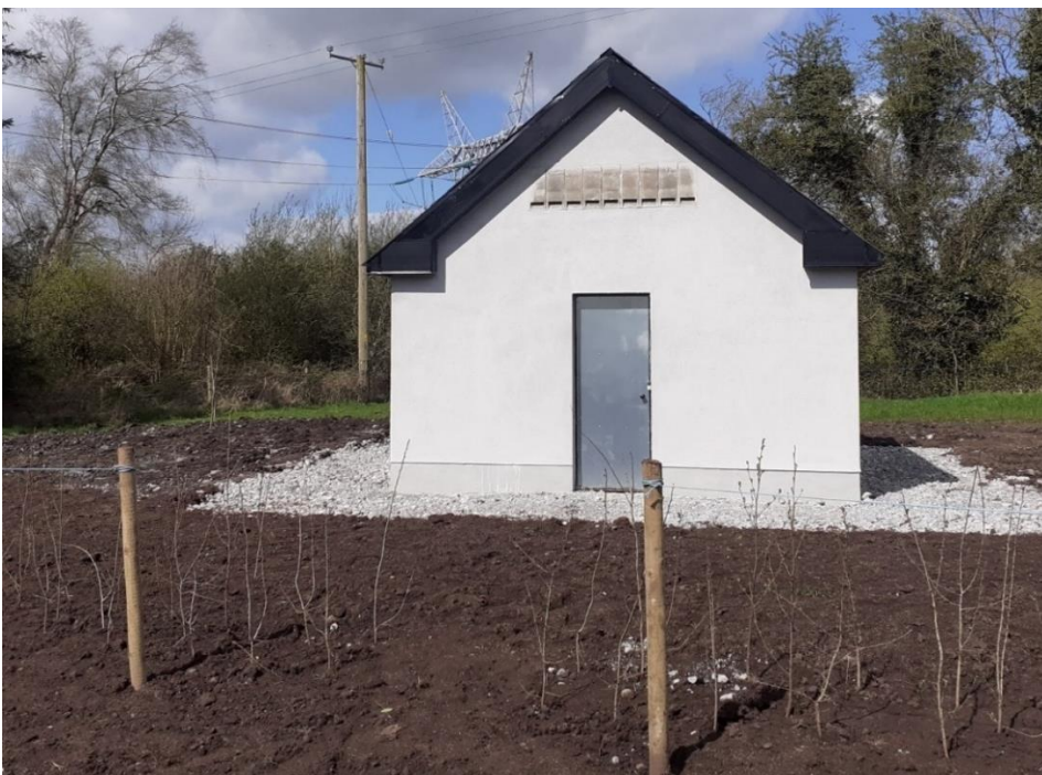
Finished look - Oldstreet Bat House (external front view with 1FR bat tubes) with boundary hedge planting.
