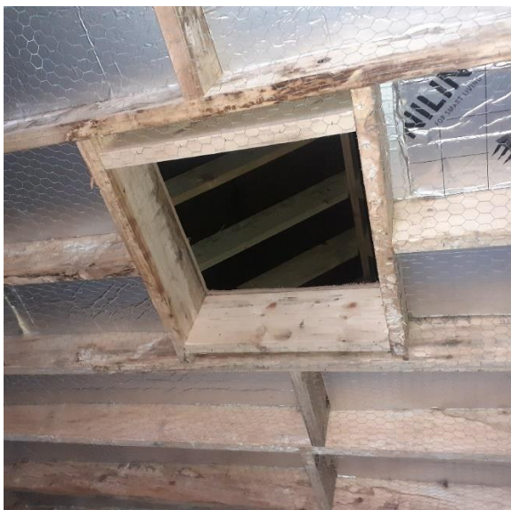
Open trap door and insulated ceiling (ground floor) of Oldstreet Substation Bat House, Co. Galway.
