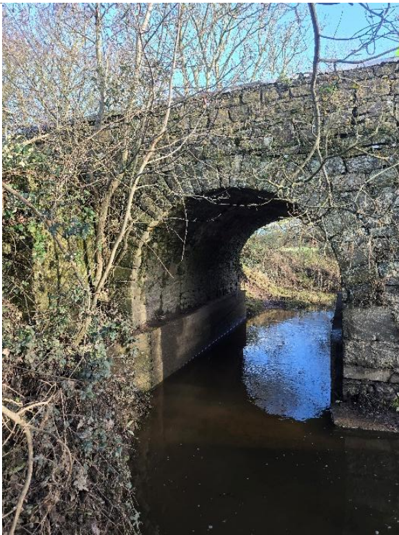
Photo 3 – General downstream elevation of third arch
