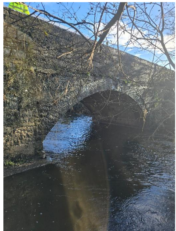
Photo 4 – General downstream elevation of central arch.
