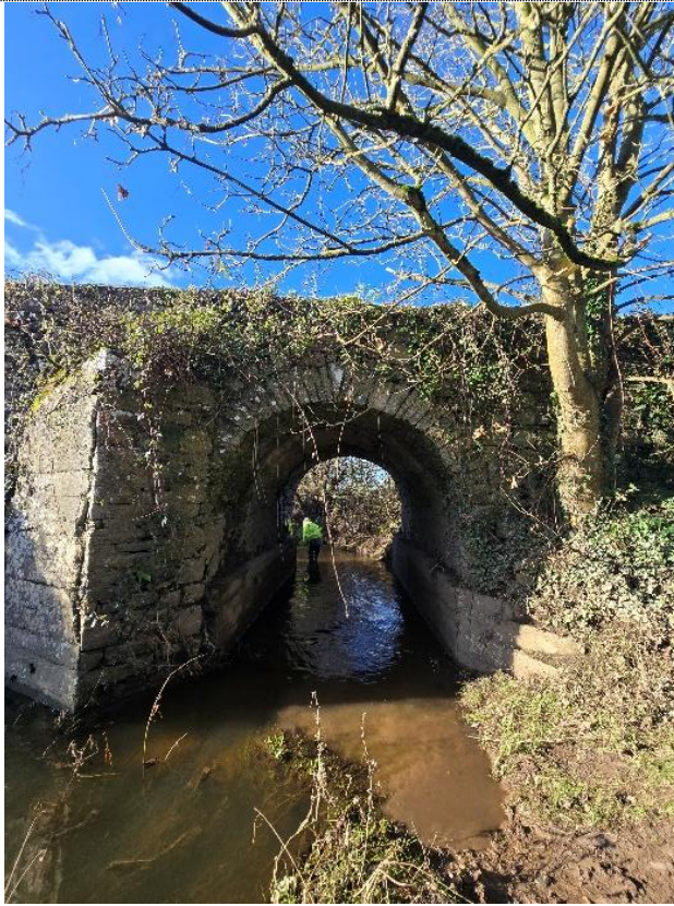
Photo 1 – General Upstream Elevation of third arch.
