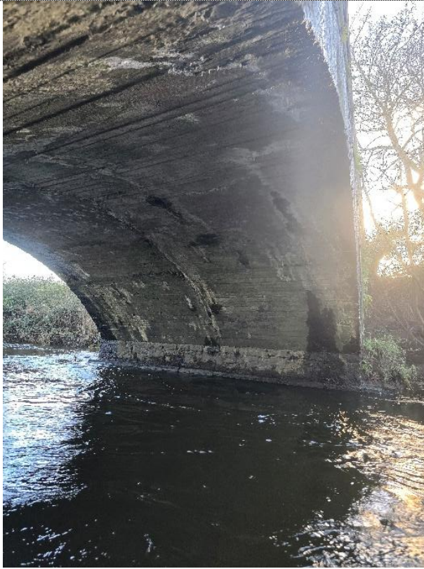
Photo 5 – General downstream elevation of central arch.
