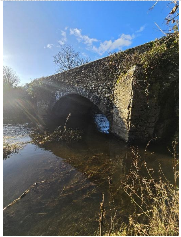
Photo 2 – General Upstream elevation of central arch.
