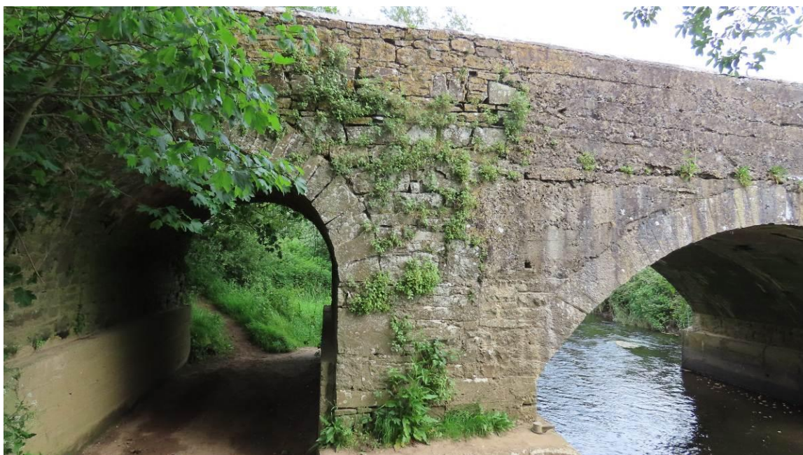
Photo 13 – northern and centre arch
