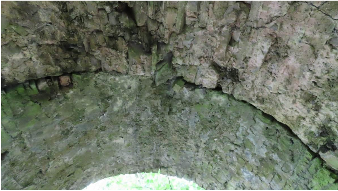
Photo 5 – joint in stonework under northernmost arch
