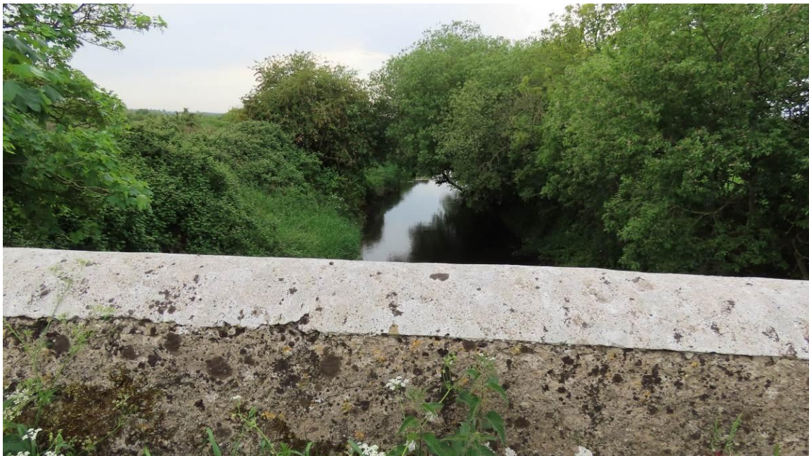
Photo 2 – watercourse upstream of bridge. Ideal foraging conditions for Daubenton's bats – sheltered still water with overhanging trees
