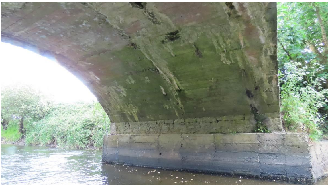
Photo 8 – undersurface of centre arch sealed with shuttered cement
