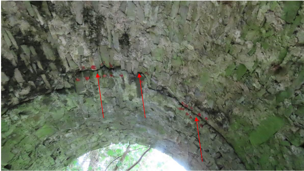
Photo 11 – sections of construction joint under southern arch marked for retention for nursery roost of Daubenton's bats
