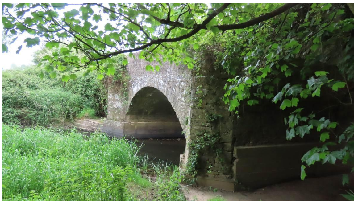
Photo 14 – looking south across bridge
