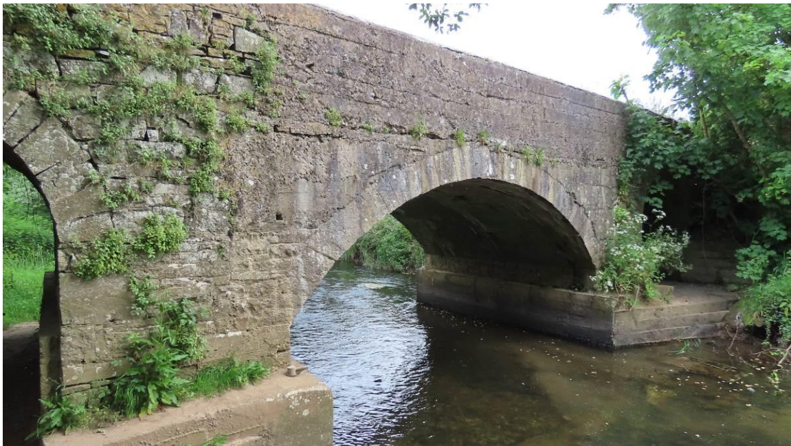
Photo 12 – upstream face of bridge showing concrete replacement parapet wall over centre arch
