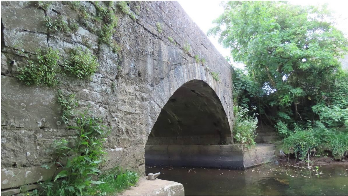
Photo 7 – looking across upstream face of bridge towards southern dry arch
