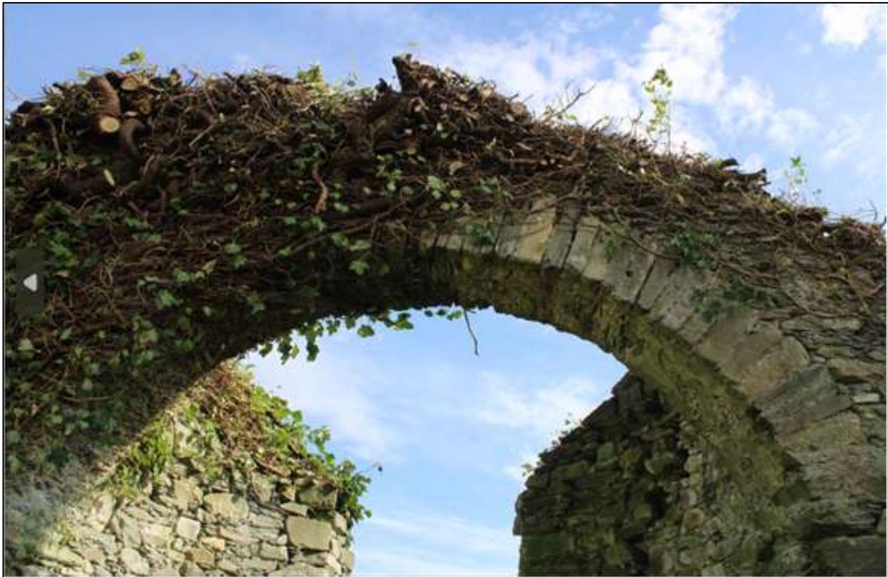
Plate 5: Voussoir construction of chancel arch.
