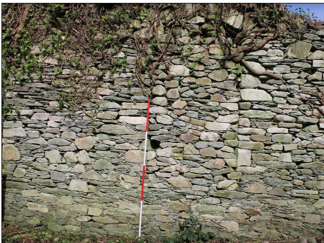
Plate 12: Blocked up window in N wall of church.
