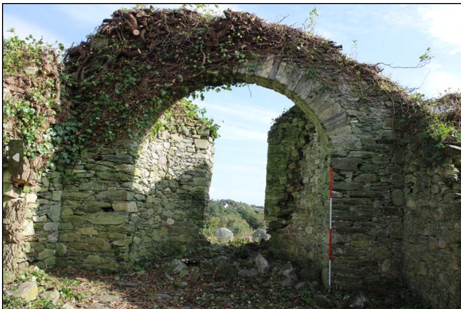
Plate 3: Chancel arch facing east.
