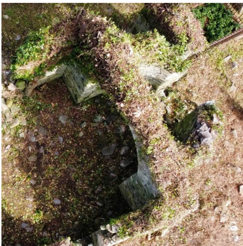
Plate 2: Overview of chancel and apsidal chamber of church.
