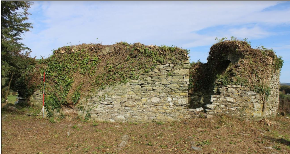
Plate 14: Southeast elevation of church.
