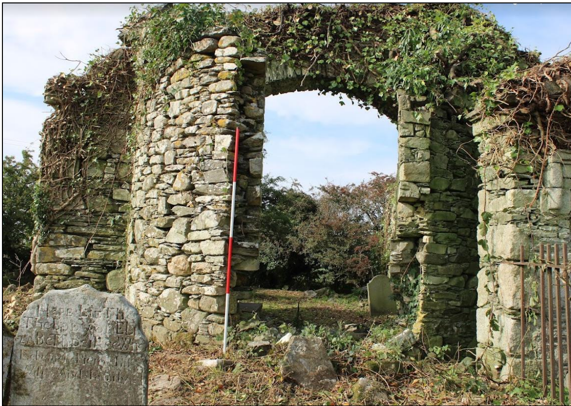
Plate 8: View of window opening in the apsidal chamber facing southwest, note how there is a small projection of masonry from the north wall.
