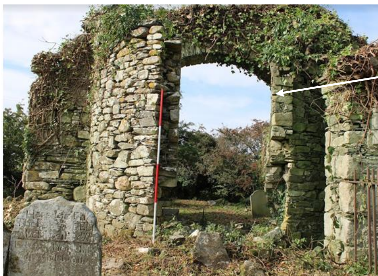
Plate 26: Trace of flat stone wall which framed the apsidal chamber as illustrated in plate 23 above.
