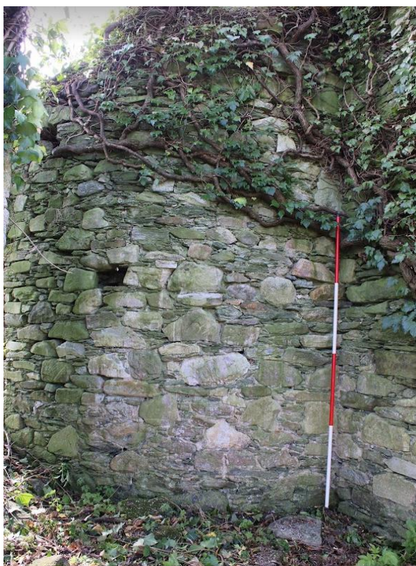
Plate 7: North wall of apsidal chamber, noted the small square hole in the wall.
