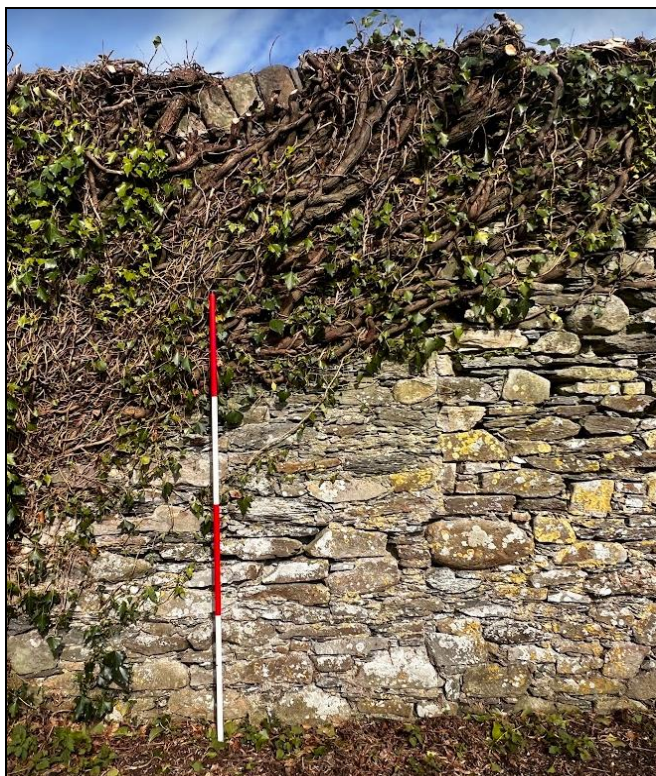
Plate 16: Blocked up window on external elevation of church.
