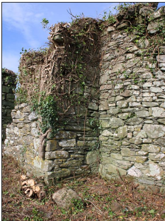
Plate 6: View of apsidal chamber and south wall of church, note how the walls appeared to have been constructed at the same time, the walls are 'knitted' together.
