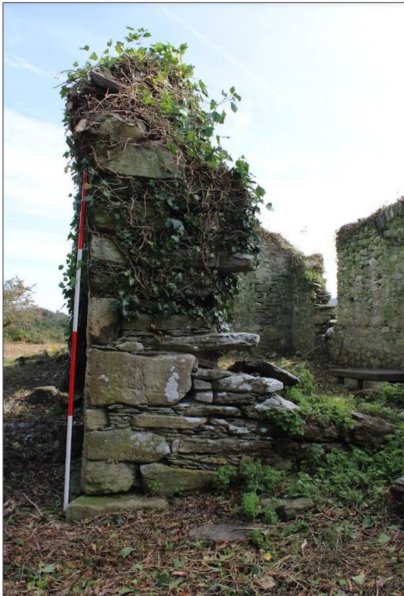
Plate 18: West view of church with sandstone quoins.
