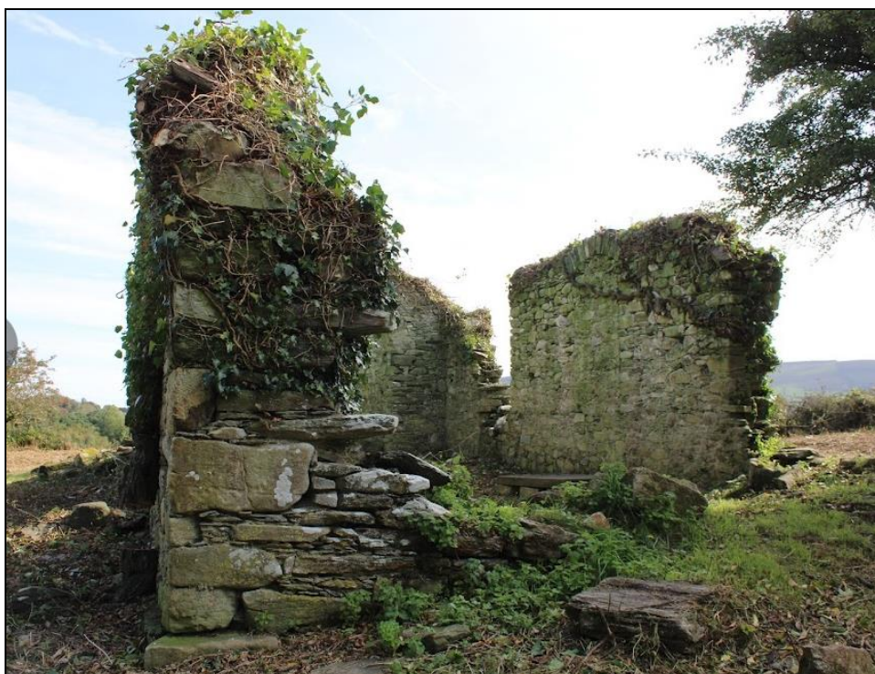
Plate 19: West gable of church.
