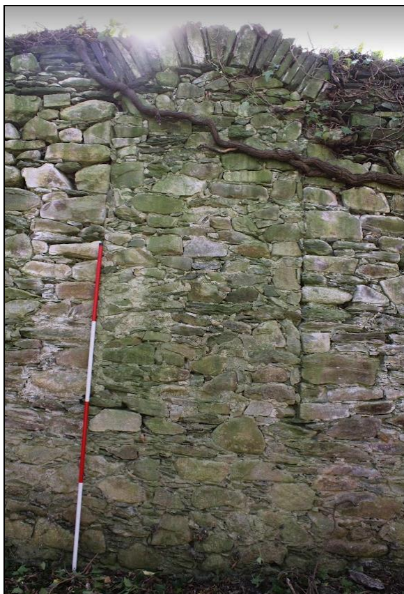
Plate 17: Central blocked up window, internal elevation of south wall of church.
