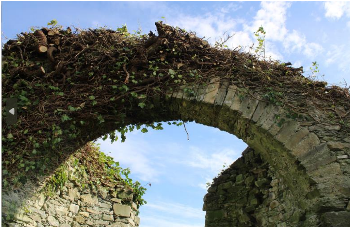
Plate 4: Voussoir construction of chancel arch.
