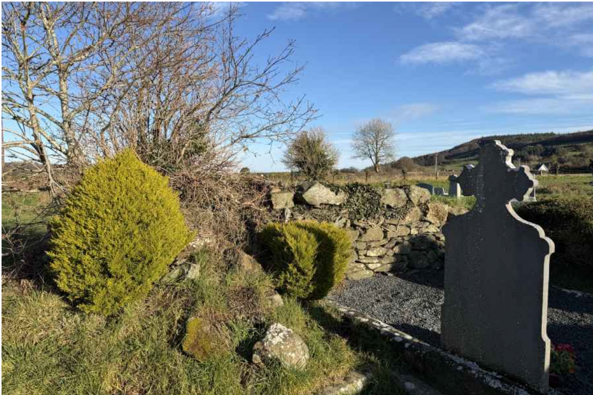
PHOTOGRAPH 15 - SECTION OF LOW SURVIVING NORTH WALL
