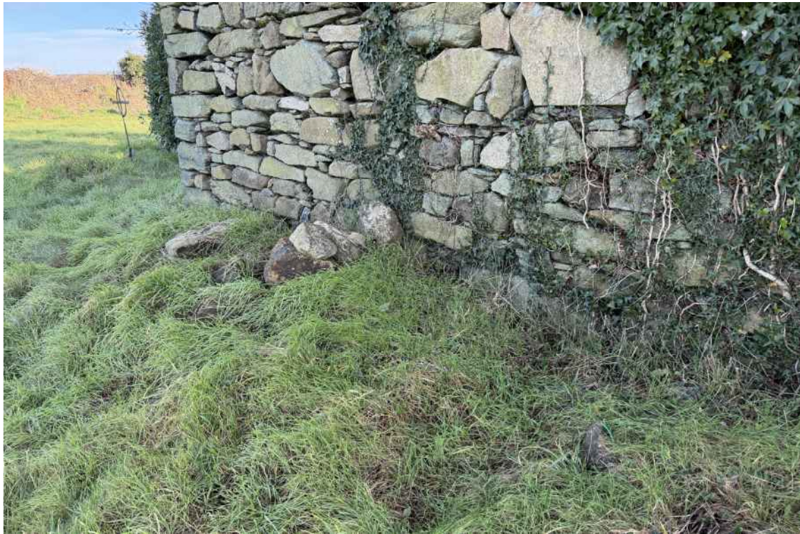
PHOTOGRAPH 5 - FALLEN MASONRY AT THE BASE OF THE WEST GABLE
