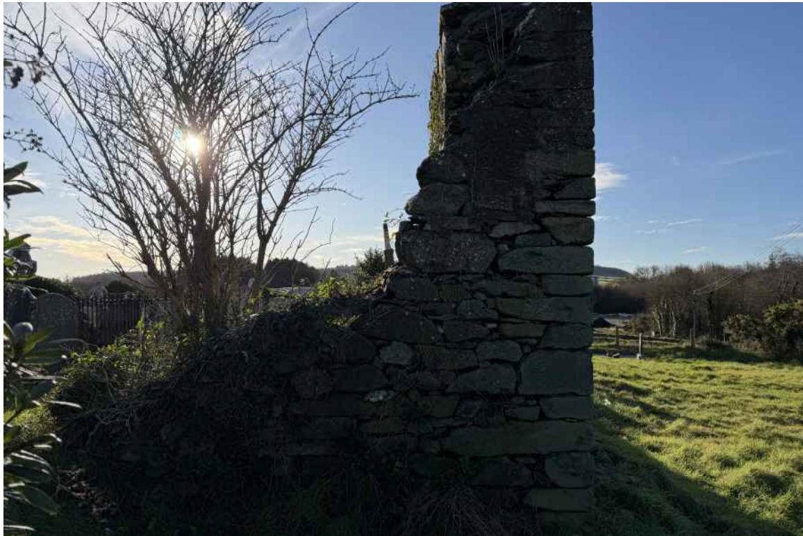
PHOTOGRAPH 7 - NORTH WALL RETURN AT THE WEST GABLE
