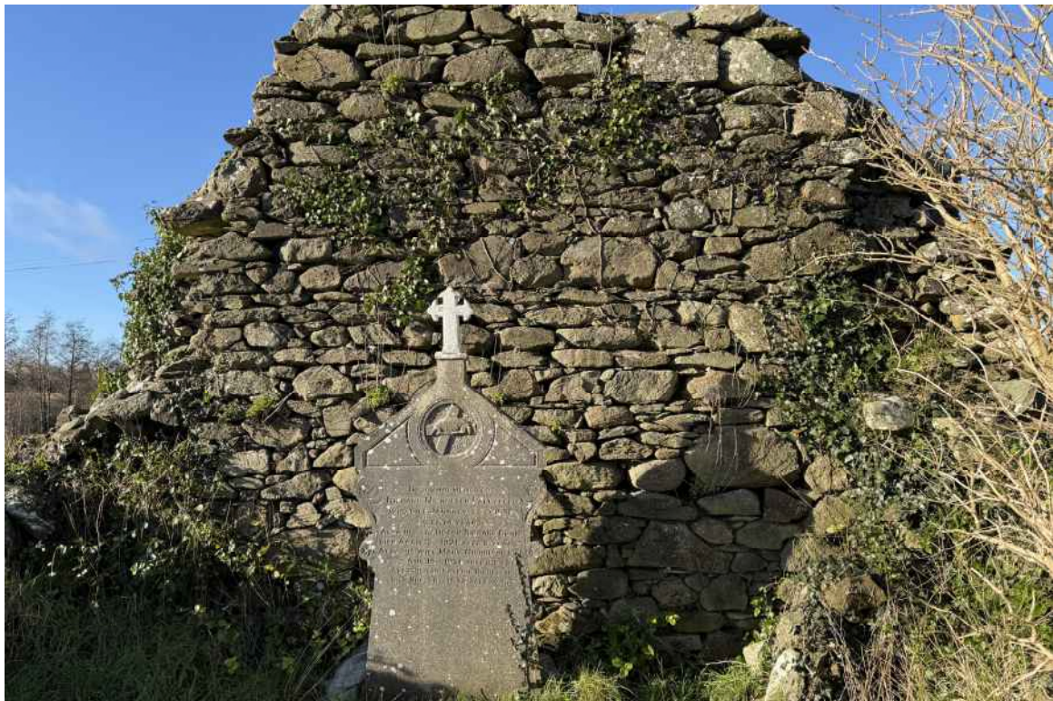
PHOTOGRAPH 10 - WEST GABLE INNERFACE
