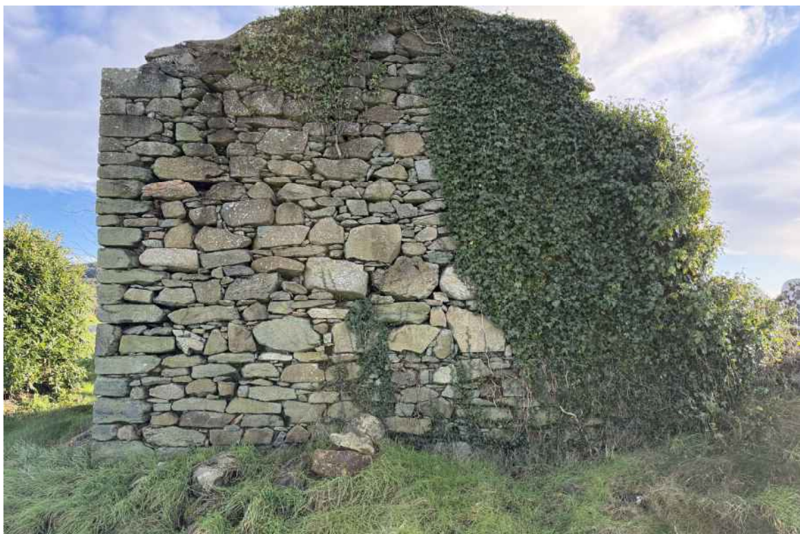
PHOTOGRAPH 2 - WEST GABLE OUTER FACE
