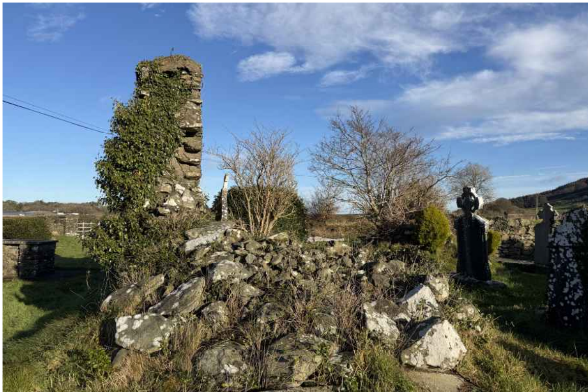
PHOTOGRAPH 6 - REMAINS OF SOUTH WALL AT THE WEST GABLE WITH COLLAPSED MASONRY STACKED AGAINST IT
