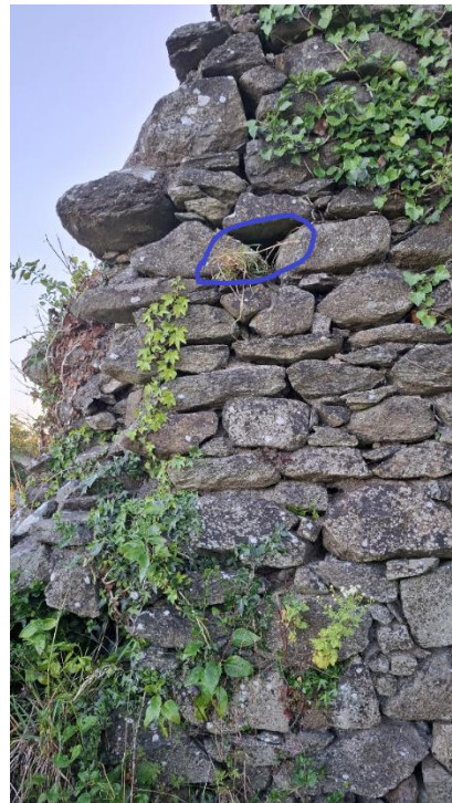
Plate 4: East side of gable wall
