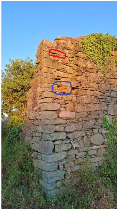
Plate 3: West side of gable wall.
