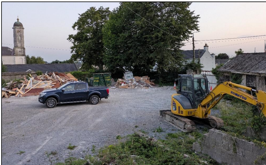
Plate 1-1. Yard containing storage buildings in southern ('lower') section of subject site.
