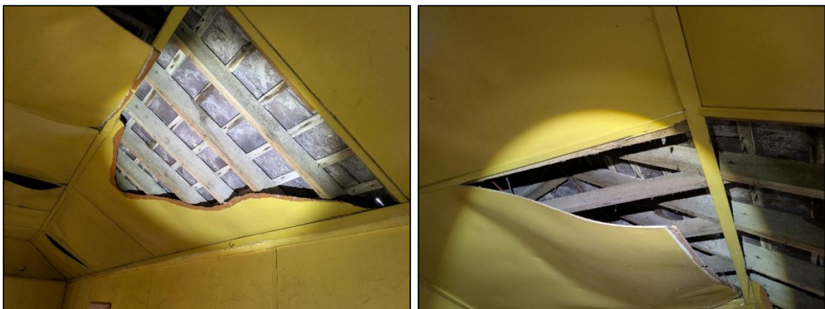
Plate 3-5. Example of attic space within Units 1-2.
