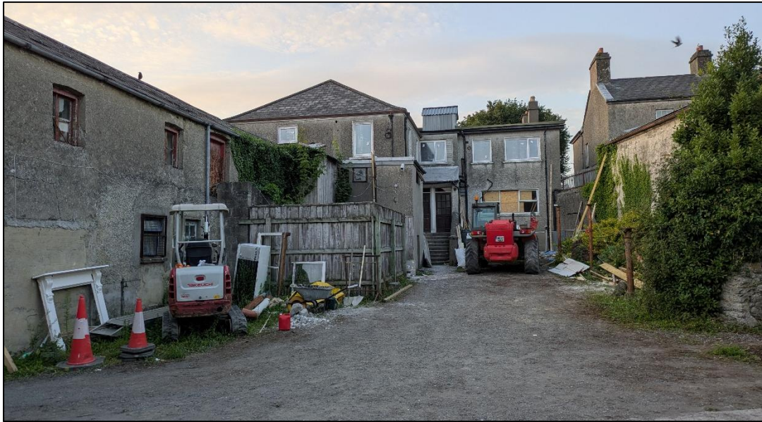
Plate 3-2. Rear of Boland's Pub and Unit 1.
