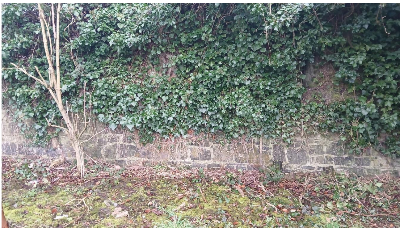
Figure 16: Removal of Ivy Side Growth from Wall
