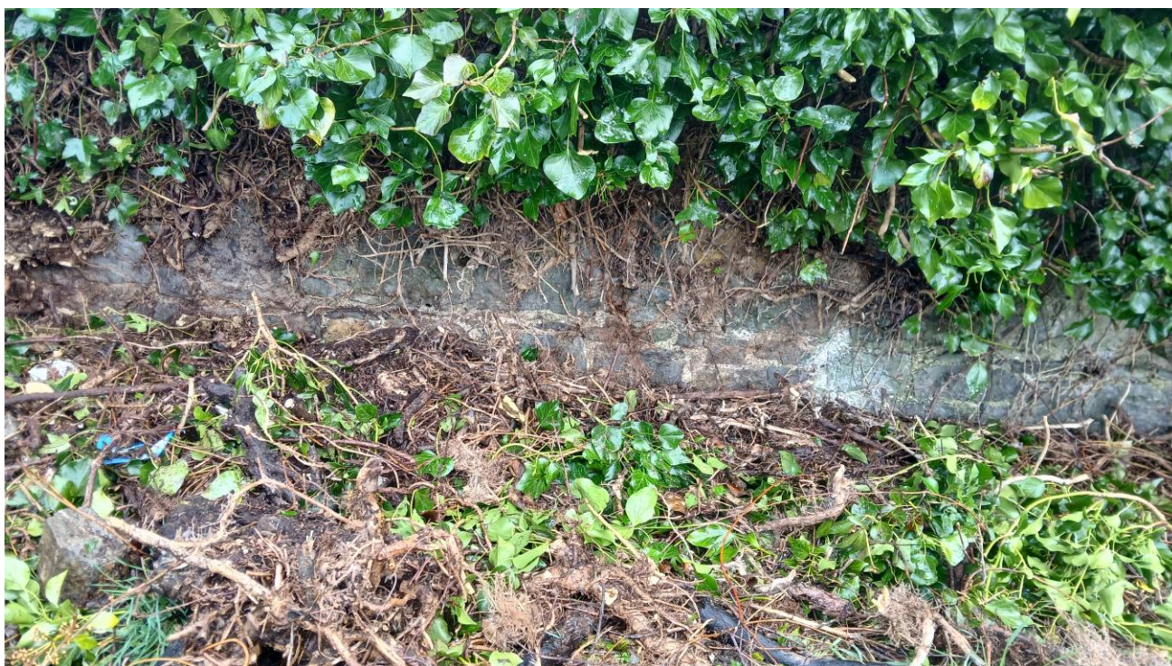
Figure 17: Removal of Ivy Side Growth from Wall
