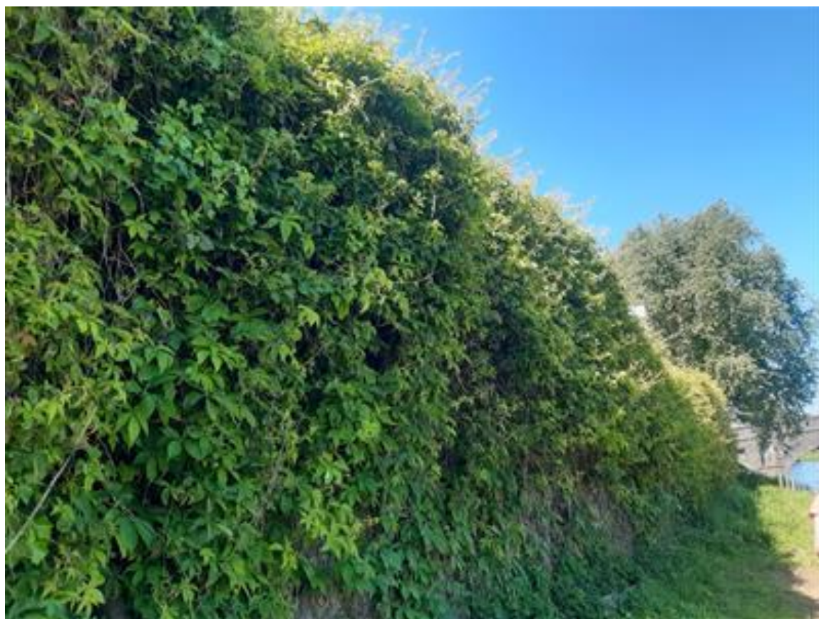
Plate 2 The wall on the eastern (i.e. Athy Marina) side showing extensive ivy and vine coverage. Note – this picture was taken prior to stem severance.
