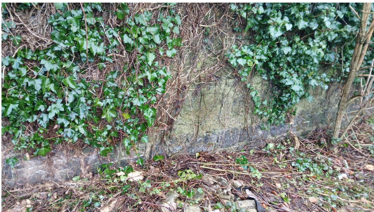
Figure 15: Removal of Ivy Side Growth from Wall
