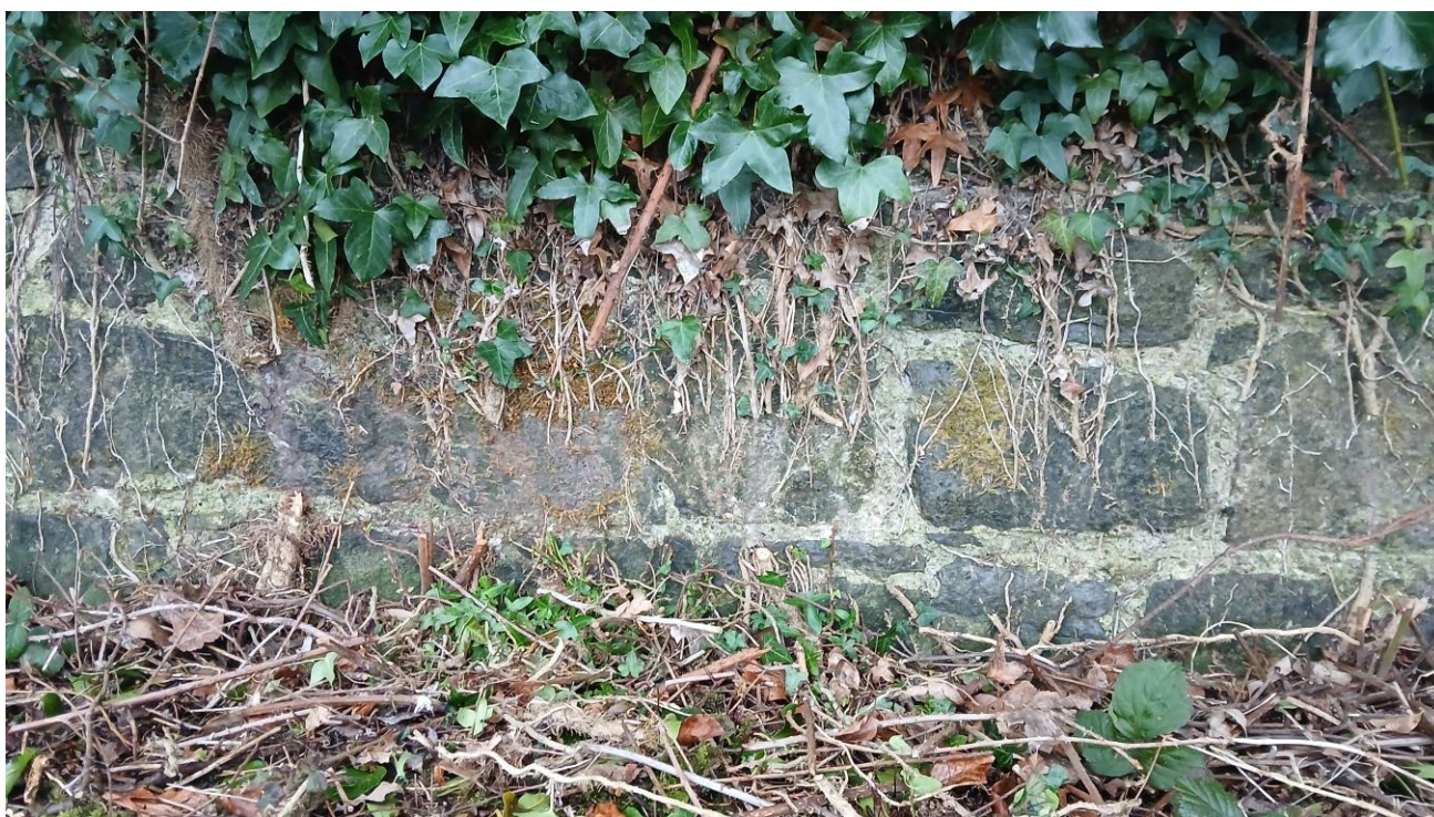
Figure 14: Removal of Ivy Side Growth from Wall
