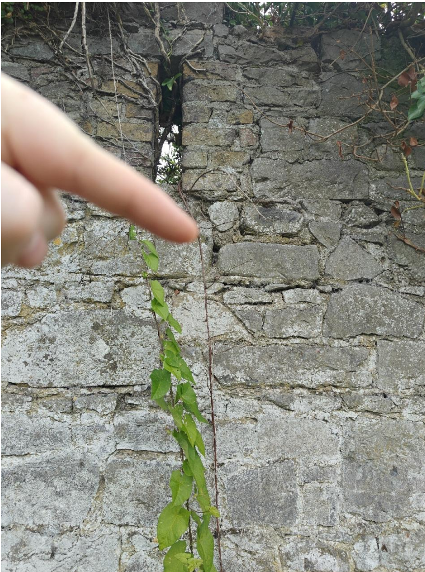
Plate 6: Location of the known bat roost (i.e. in the gap in the stonework being indicated by the surveyor)
