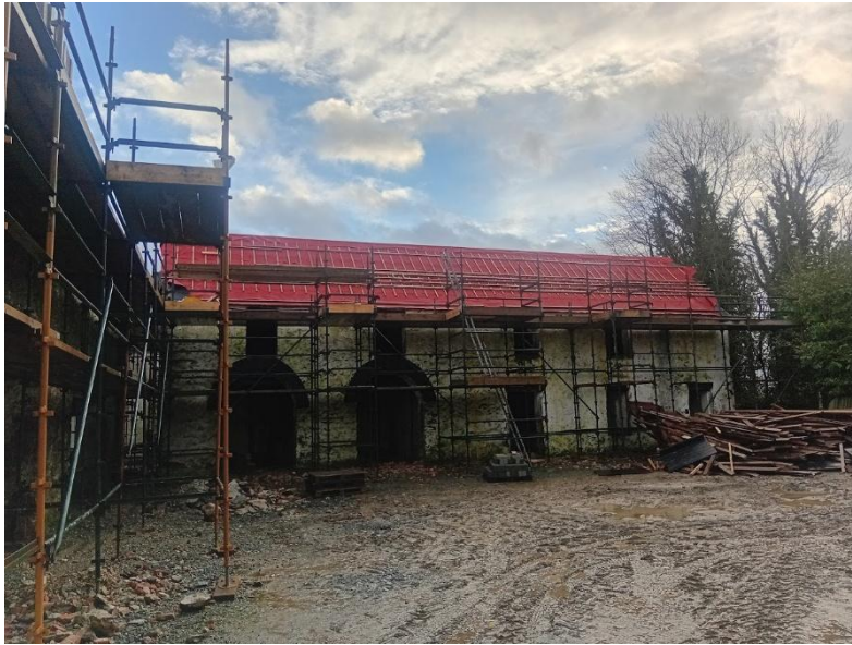
Roof exterior Stable A
