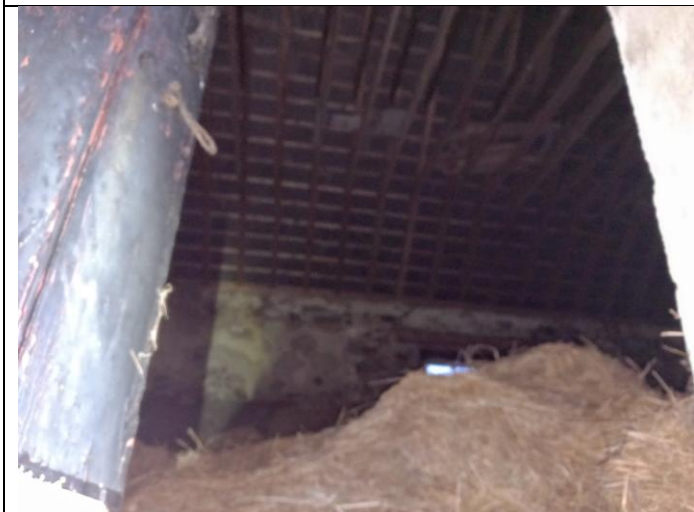
Interior of loft space Stable B
