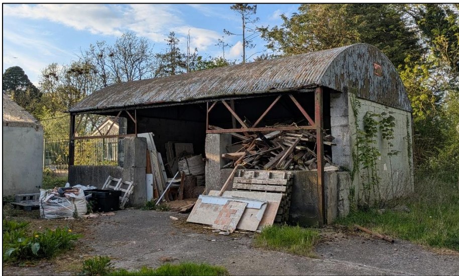
Plate 3-6. Building 'B3' within proposed development site.
