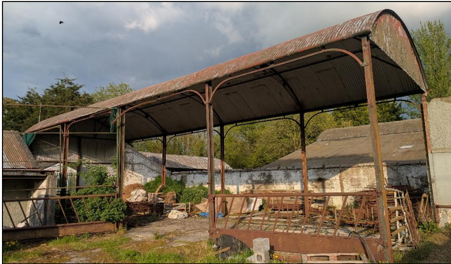
Plate 3-5. Building 'B2' within proposed development site.
