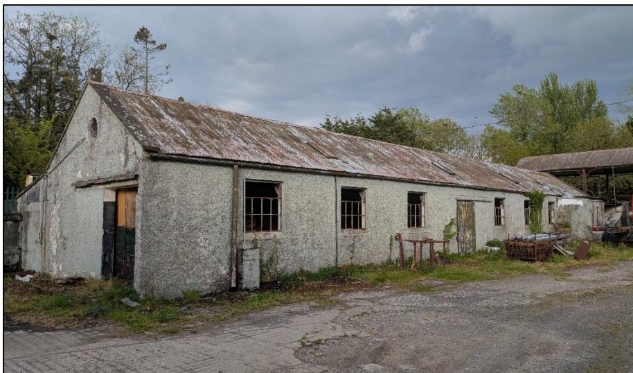
Plate 3-1. Building 'B1' within proposed development site.
