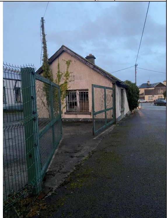
Plate 9: western view of the southern building
