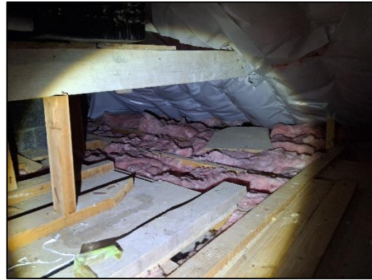
Plate 5-2 Attic with underfelt lining and loft insulation
