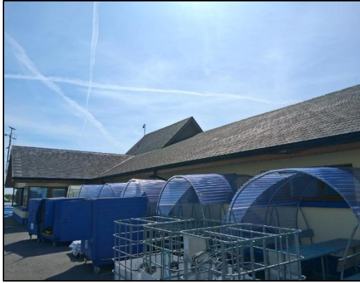
Plate 5-1 Exterior view of the BaySports building
