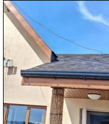
Plate 5-2 Potential access points identified during the exterior inspection
