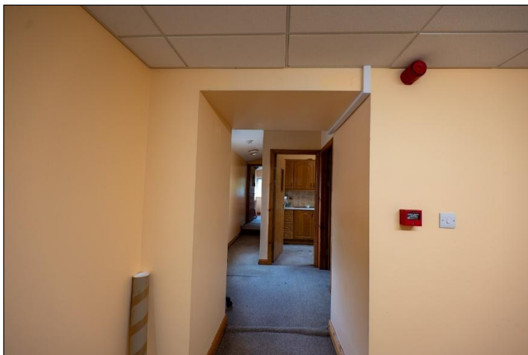
Plate 4 Internal inspection of subject building.
