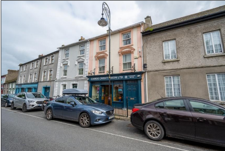
Plate 1 The subject Cairde Credit Union Site, viewed from the front of the building.
