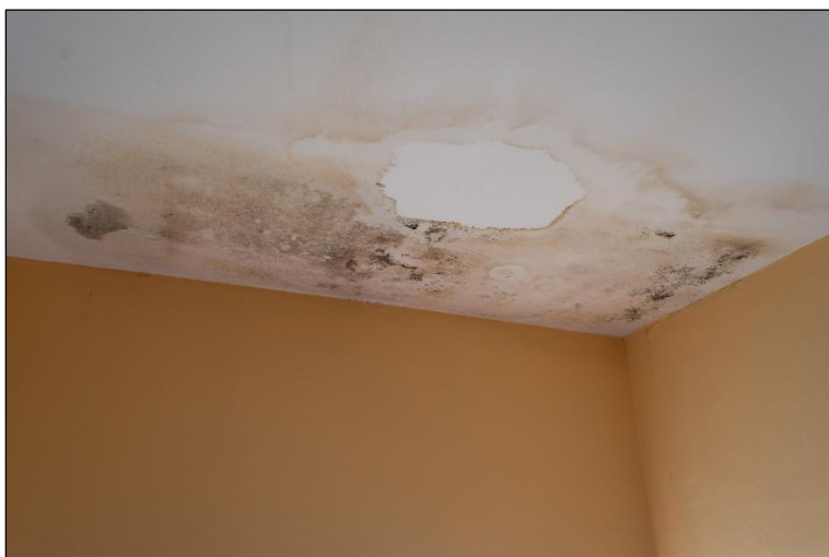
Plate 5 Internal inspection of subject building.
