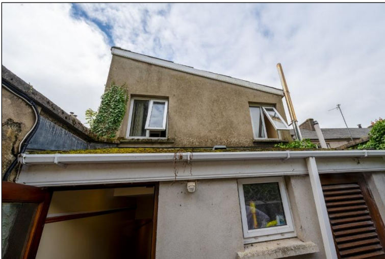
Plate 2 The subject site, viewed from the rear.
