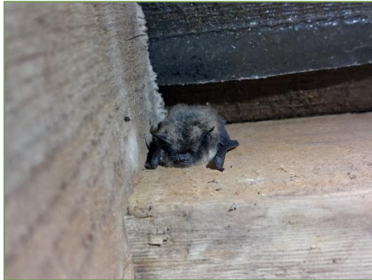
Plate 3.1 Whiskered Bat roosting along the ridge beam within the western attic section of Lissardagh House.
