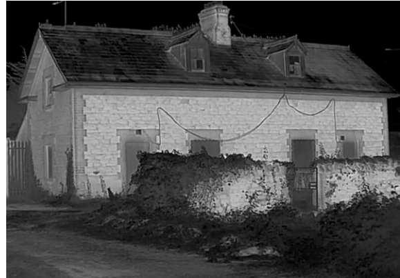
Plate A2. Thermal camera still image showing the west and north elevations.
