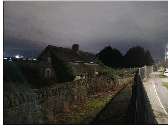
Plate 14. Building exterior rear and side (east and south elevations). Ballycoolen Road on right
