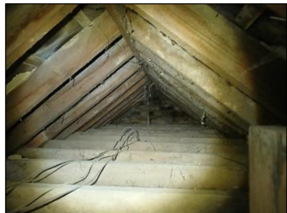
Plate 10. The roof is unlined, with the underside of the slates exposed. Attic shows no signs of bats
