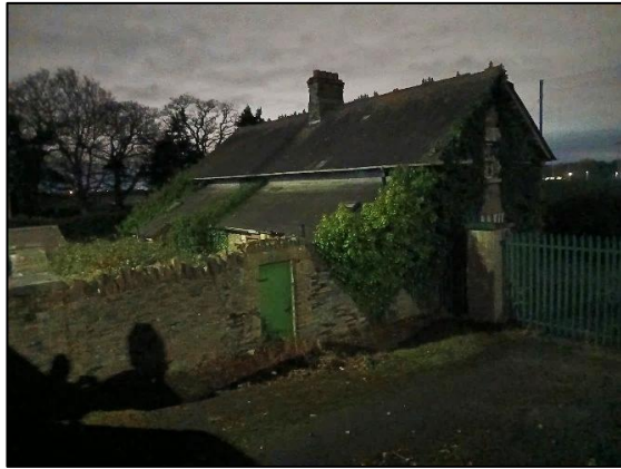
Plate 13. Nighttime view of building exterior, rear and side (east and north elevations). The building is subject to significant light pollution from the adjacent street lighting on Ballycoolen road.
