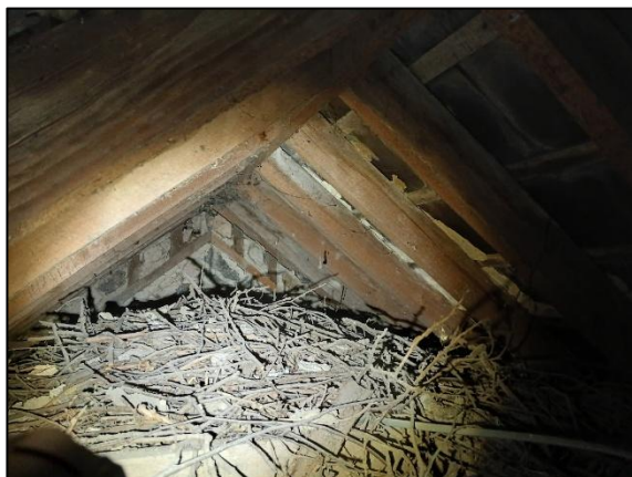
Plate 9. Historic signs of birds nesting noted: roof has been repaired in recent years, no signs of bats or birds observed
