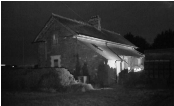
Plate A3. Infra-red camera still image showing the south and east elevations at end of dusk emergence survey
