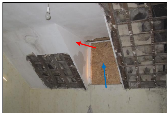
Plate 6. Interior of first floor room with boarded up dormer window (blue arrow) and approximate location of roost (red arrow)
