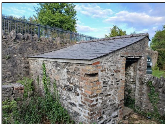
Plate 11. Southern outhouse. No signs of bats noted. Outhouse interior lacks the structural elements which would provide suitable roosting areas for bats with a lack of crevices and shelter from light and draughts. A single barn swallow's nest was recorded on 6 th May 2026
