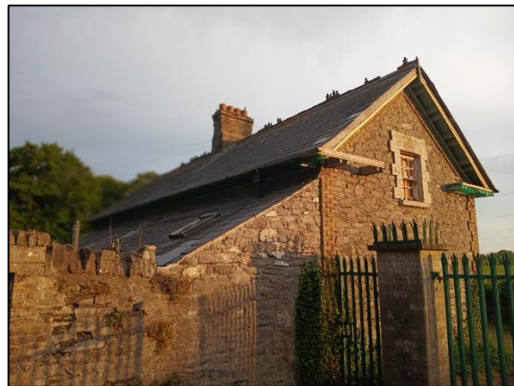
Plate 4. East elevation (left) and north elevation (right)
