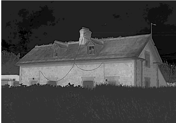
Plate A1. Thermal camera still image showing the west and south elevations
