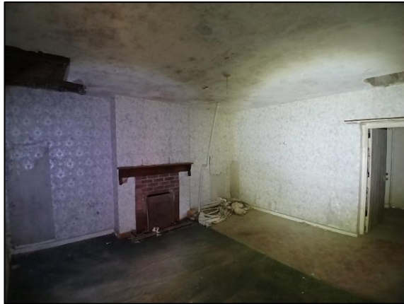
Plate 7. Ground floor room, windows have been shuttered
