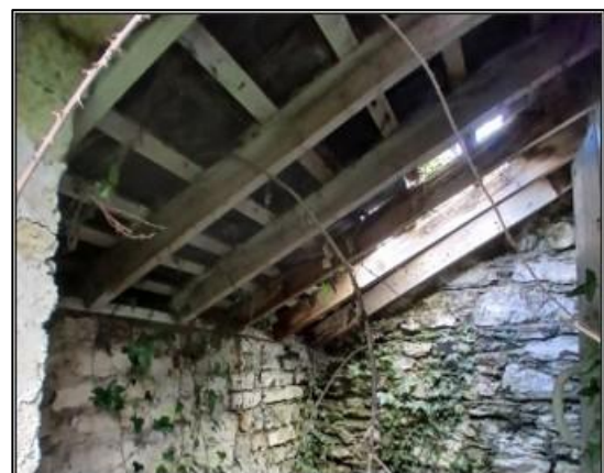
Plate 12. Northern outhouse interior. No signs of bats noted. Outhouse interior lacks the structural elements which would provide suitable roosting areas for bats with a lack of crevices and shelter from light and draughts
