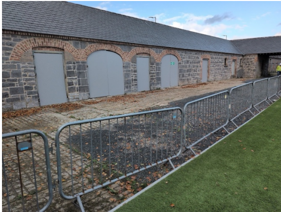
Plate 3. Existing Courtyard buildings
