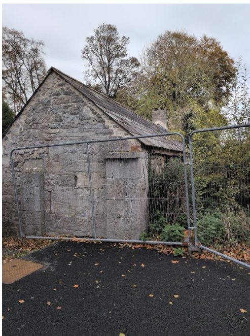
Plate 6. Exterior of building 12
