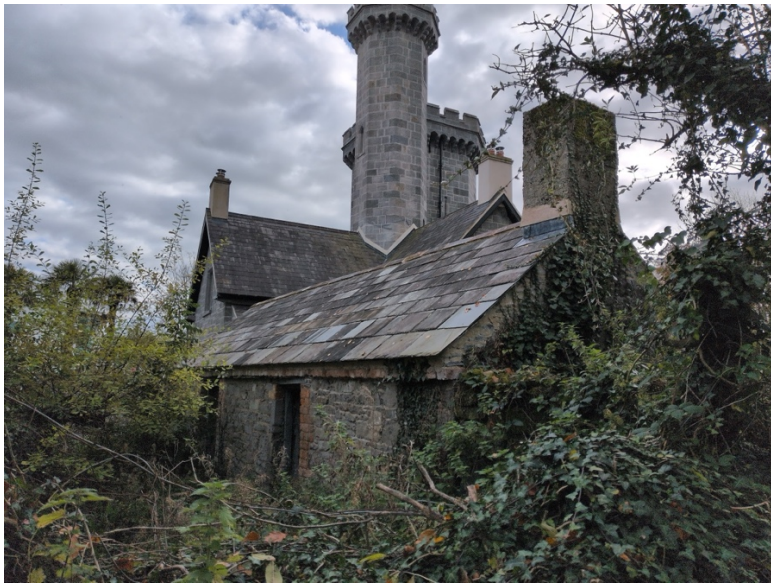
Plate 5. Exterior of building 12
