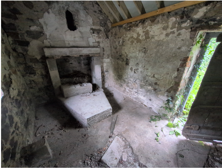
Plate 3. Interior of Room 2. Chimney structure within room 2 to be capped, internal structure will be cleared of old corvid nests to provide potential bat habitat. Door to be modified to prevent drafts of light spillage.
