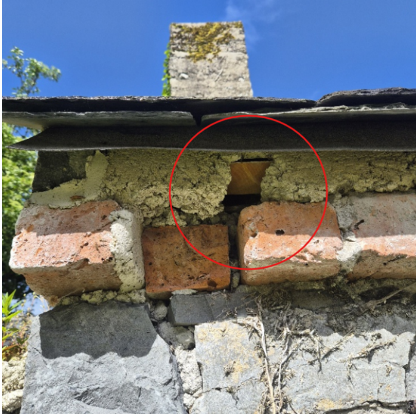
Plate 5.Existing opening on Building 12
