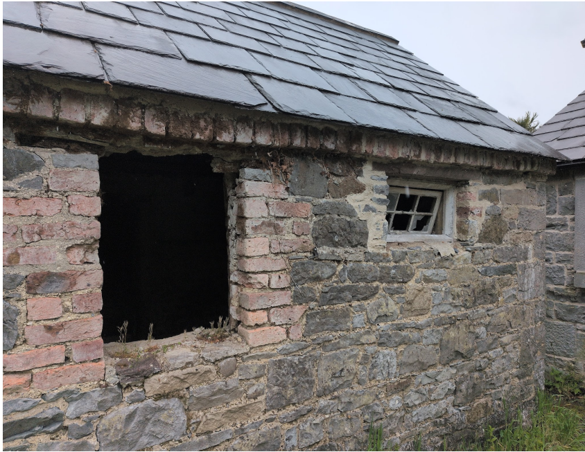
Plate 1. Exterior of room 1: This window to be modified to create access point for lesser horseshoe bat via a 50cm x 50cm gap (with a cowl lead will be used to prevent predator access). The smaller windows will be blocked with plywood. Small gaps along the base of the walls will also be blocked to prevent rodent access.
