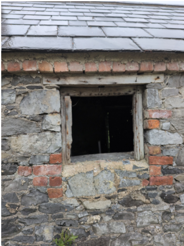
Plate 4. Exterior of room 2: Window to be blocked with plywood. The objective for room 2 is to minimise draughts and light spillage and provide suitable conditions for Lesser Horseshoe bat roosting
