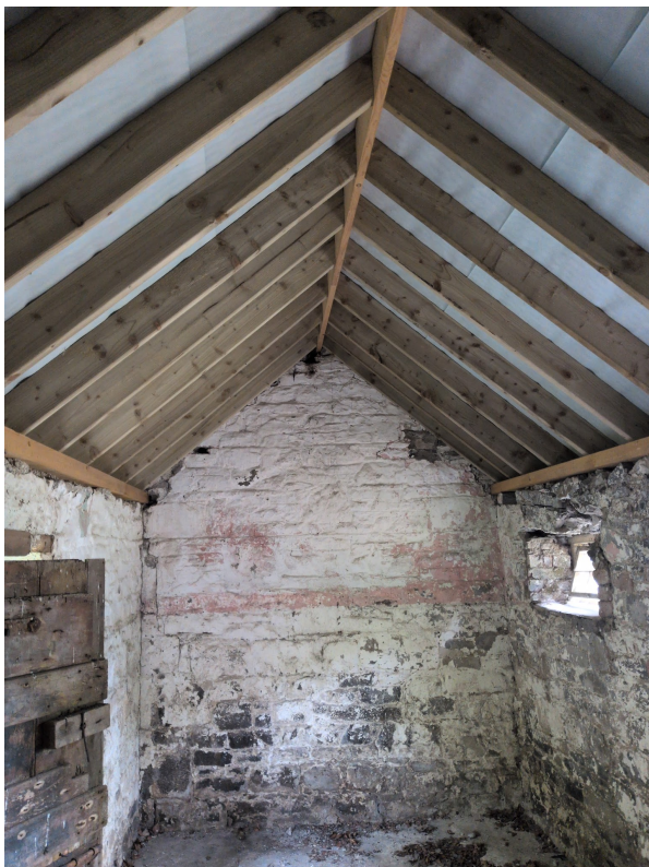
Plate 2. Room 1 interior. Location of loft space on gable wall. Door to be replaced/sealed.
