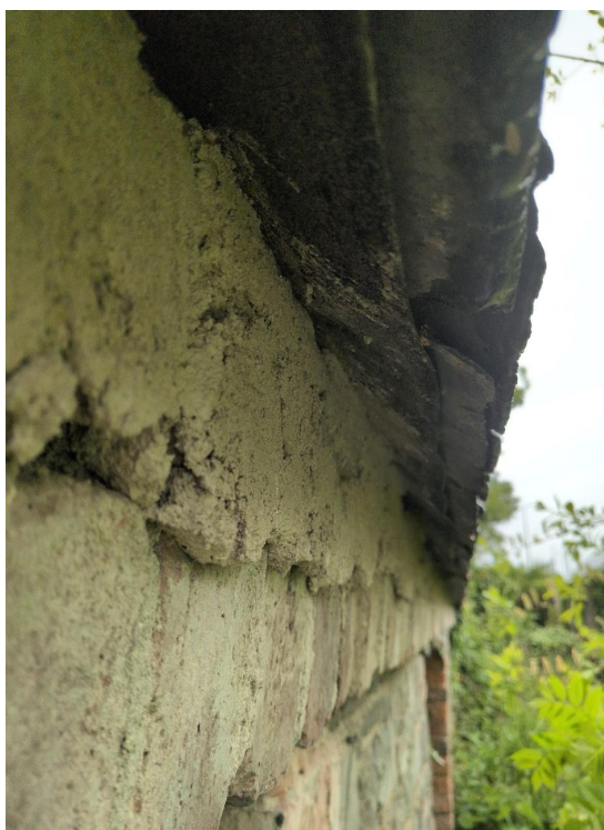
Plate 6. Closer view of concrete fill. This will be removed in part to allow gaps
