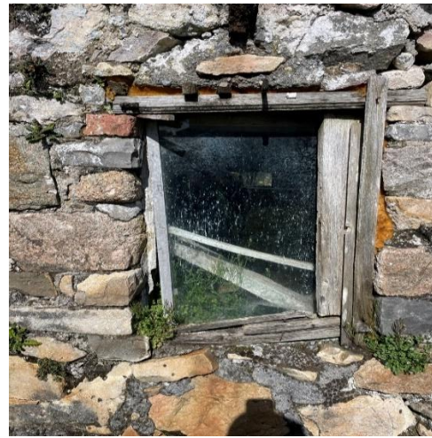
Plate 5-2 Access through the window
