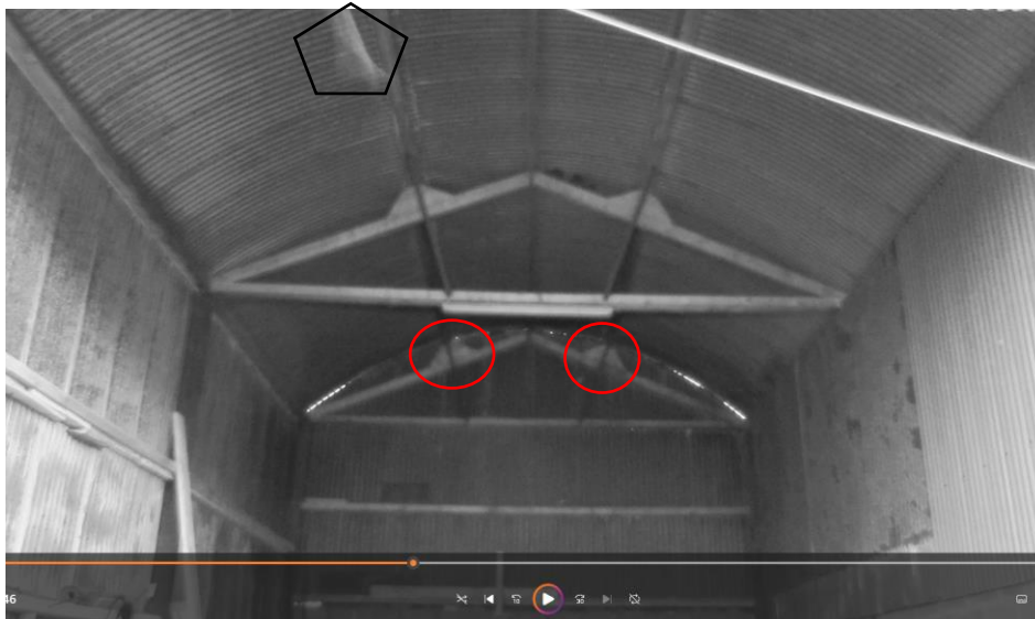
Fig 9: Location of roosting bats at the hay barn in Cliffony. Leisler's on the left and Soprano Pipistrelle on the right. See the blurred still, captured from video footage of the emerging Leisler's bat. 🏠
