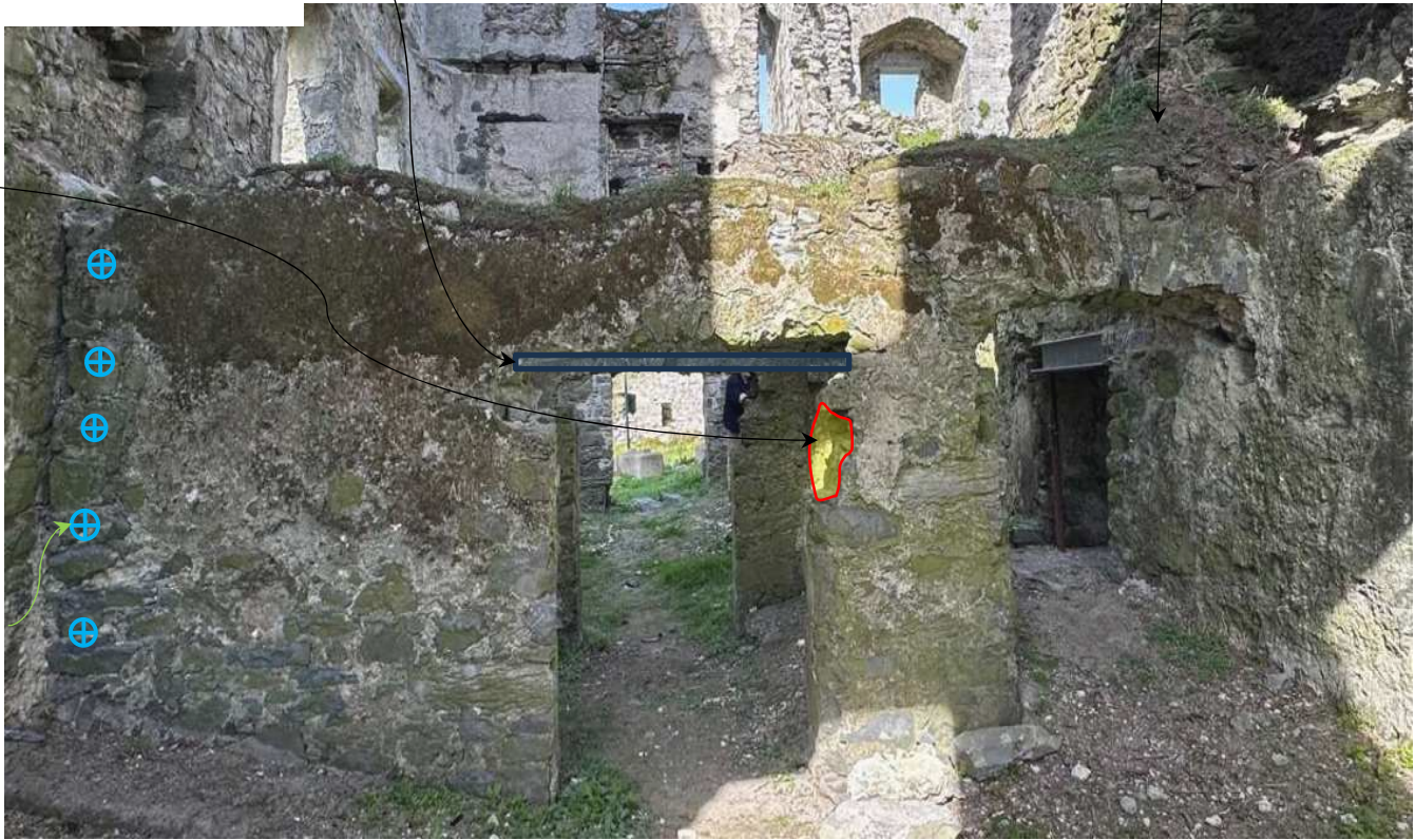
INTERNAL WALL 1 - LOOKING NORTH
