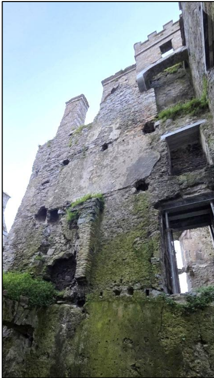
Plate 1: West side of internal spine wall to be repaired as part of Phase 6
