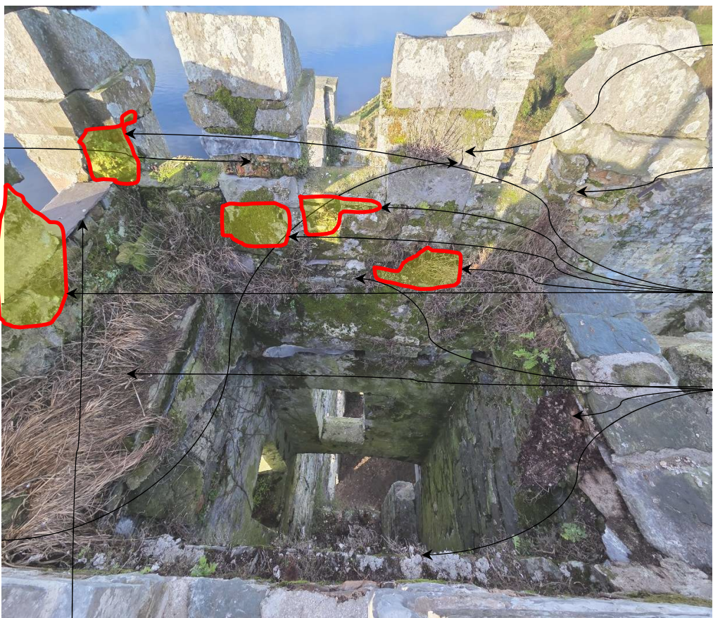
INTERNAL WALL LOOKING SOUTH & WEST
