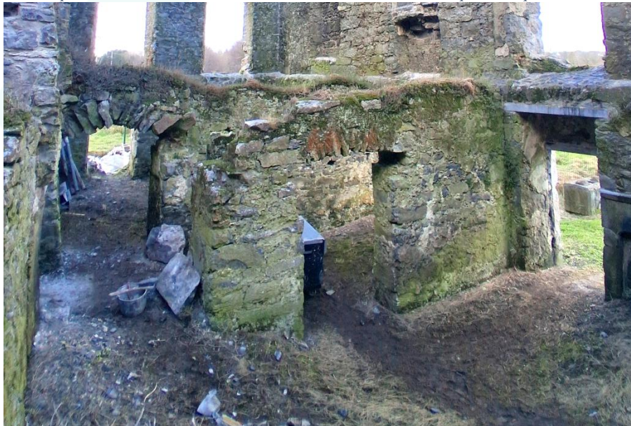
Plate 3: Internal ground level walls in the west area of the castle to be repaired as part of Phase 6
