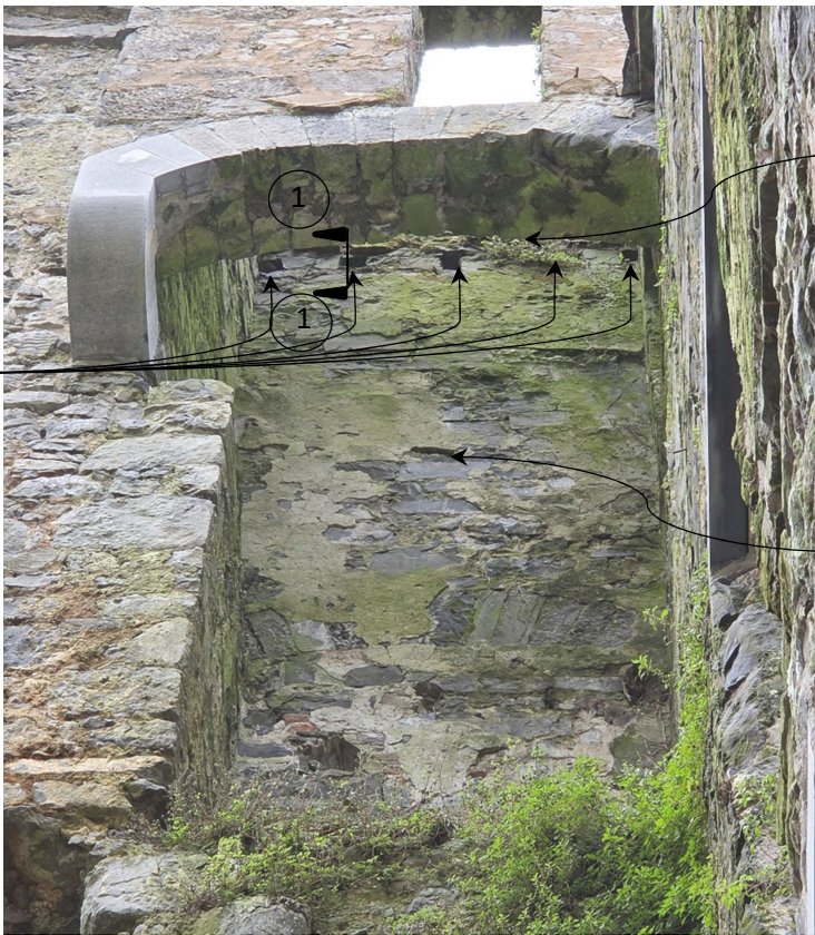
INTERNAL WALL LOOKING EAST
