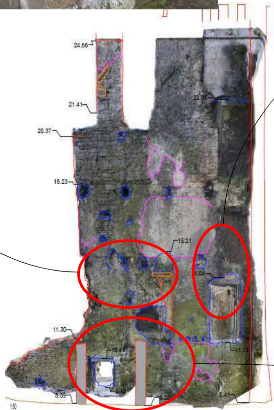
INTERNAL WALL LOOKING EAST
