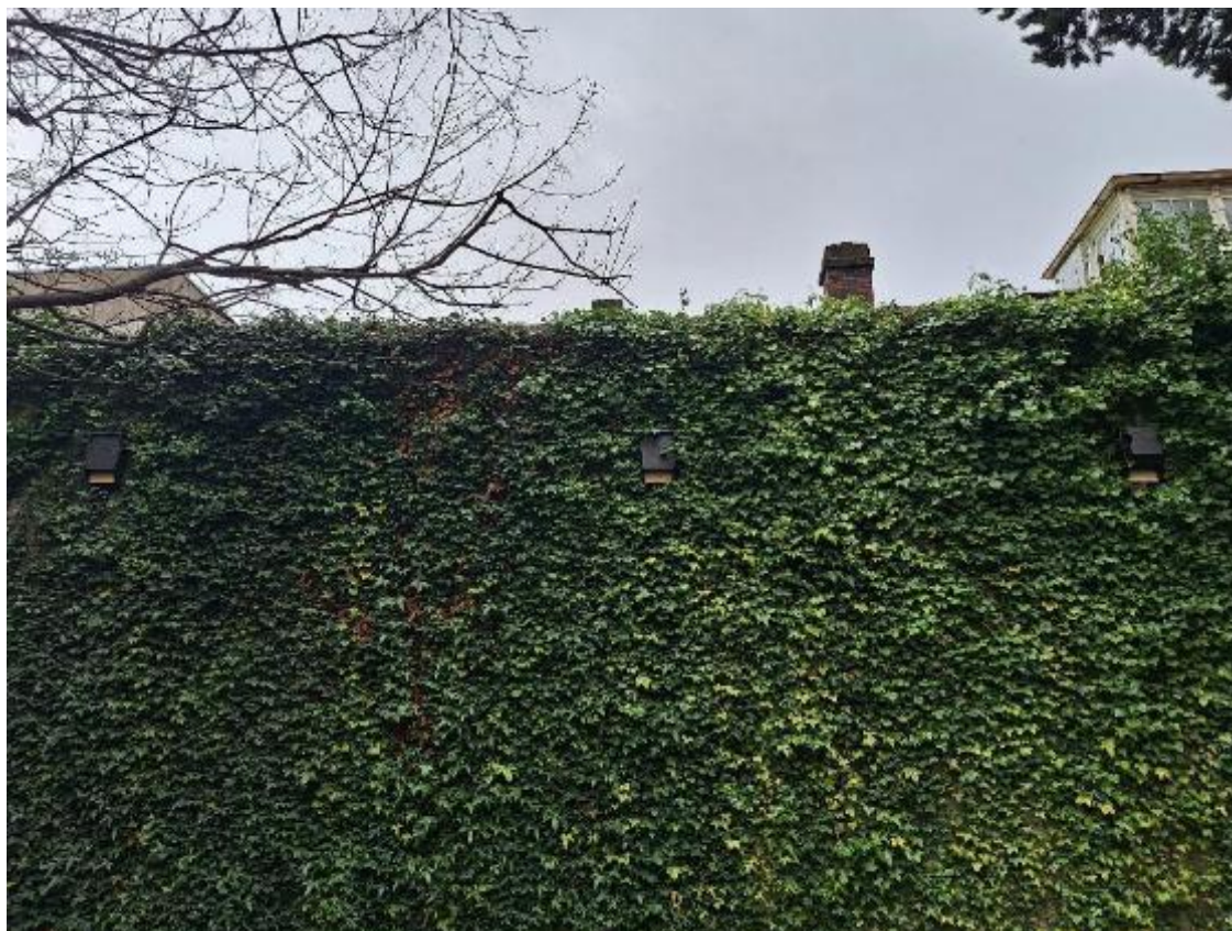
Plate 2. Bat Boxes installed as mitigation in the Iveagh Gardens
