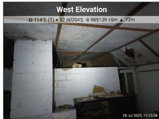
Plate 3.4 Interior view of northern main section, showing enclosed attic space.
