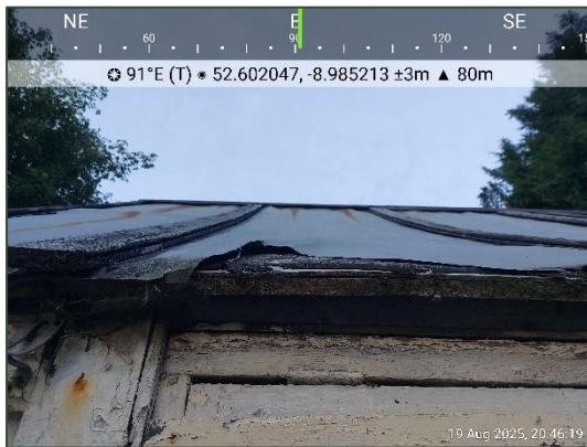
Plate 3.3 View of lead roofing of southern adjoining section.
