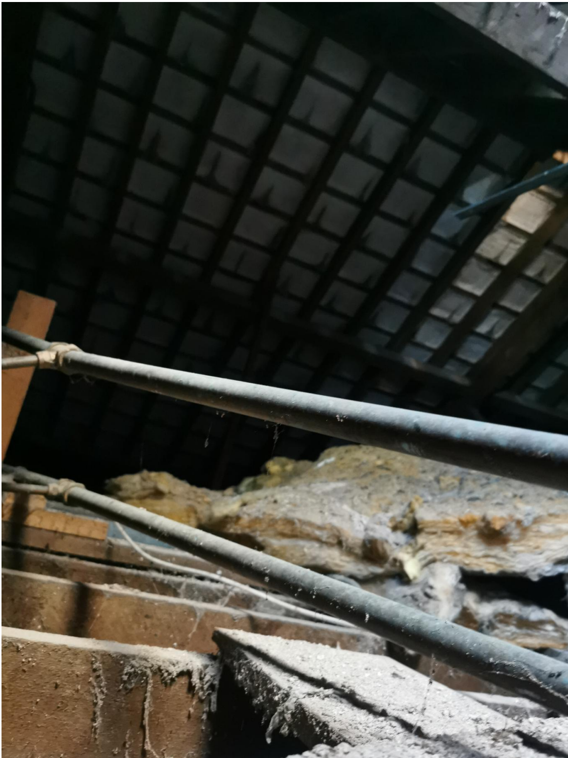
Figure 4-11: East wing attic
