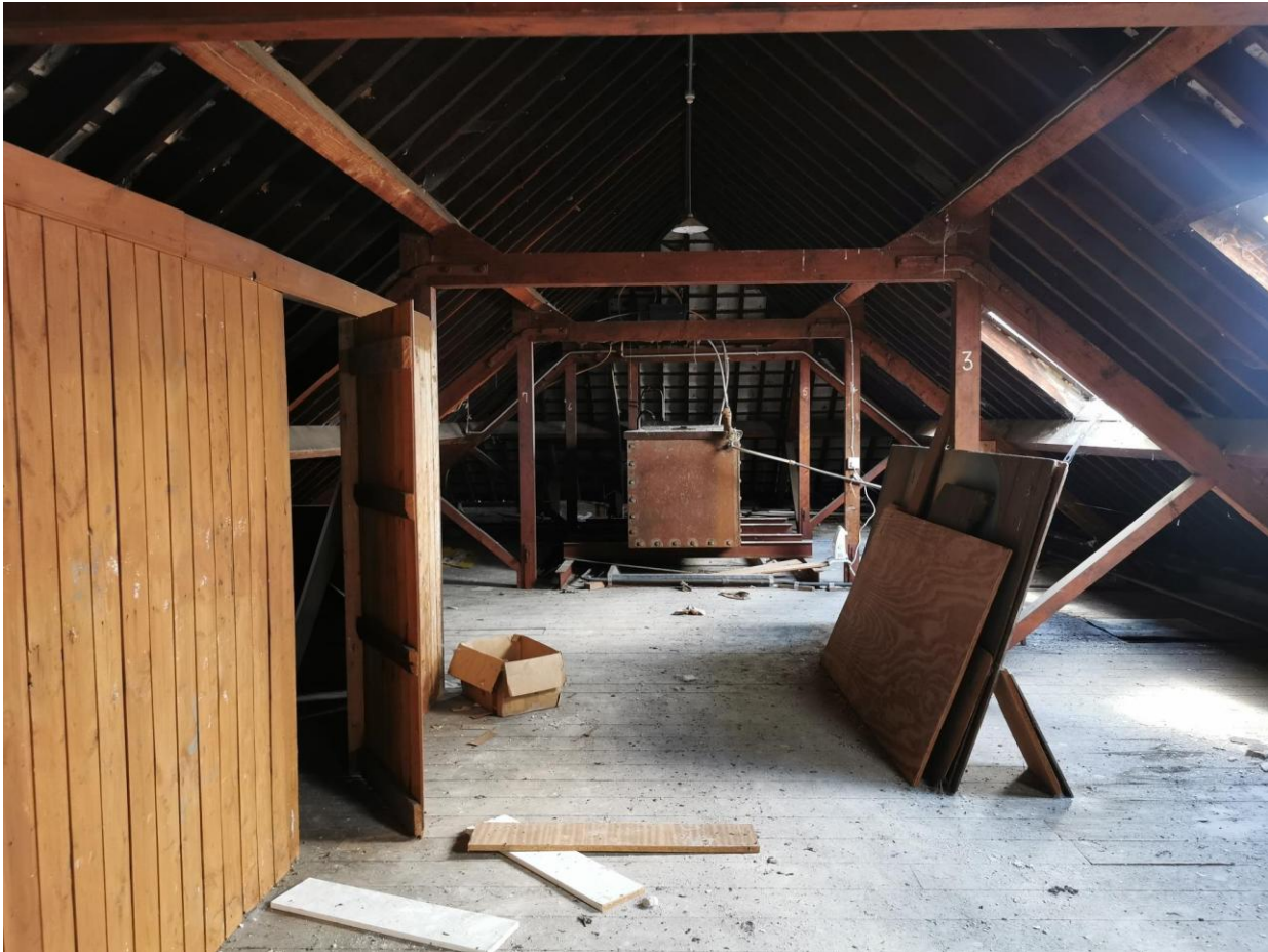
Figure 4-7: West wing attic
