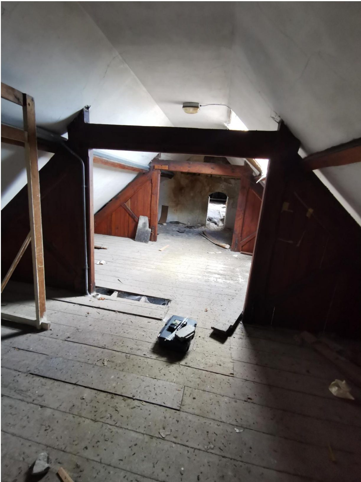
Figure 4-8: Central attic space
