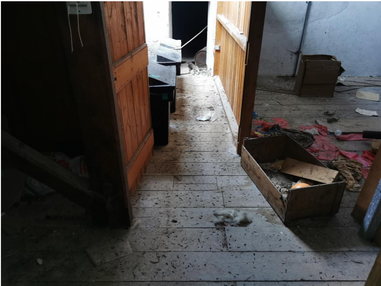
Figure 4-9: Central attic space (main roost location in dark area visible in image background)
