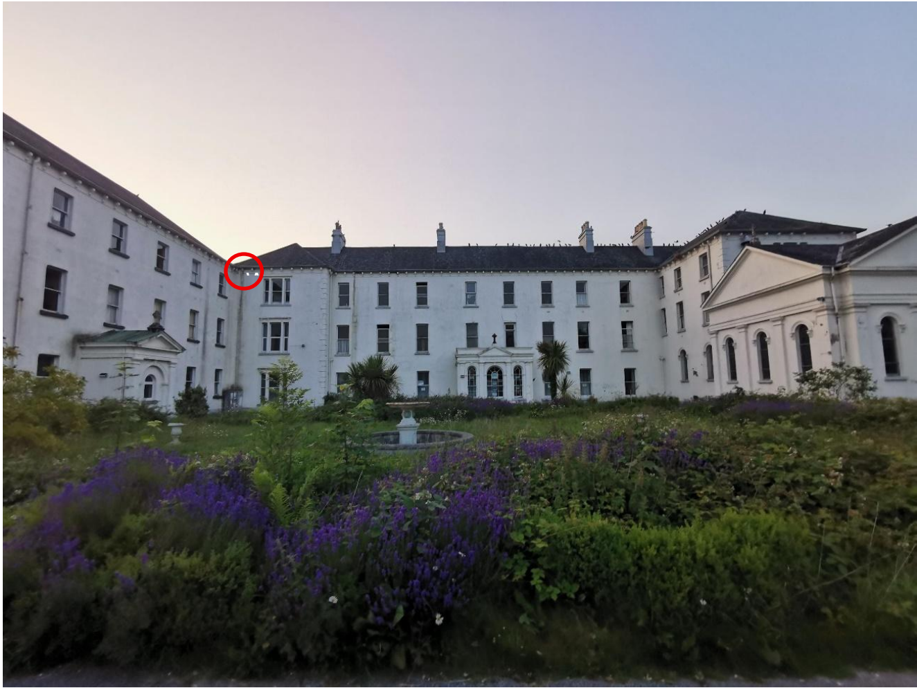
Figure 4-5: Emergence points for Common Pipistrelle from southern face of convent building (18 June 2025)
