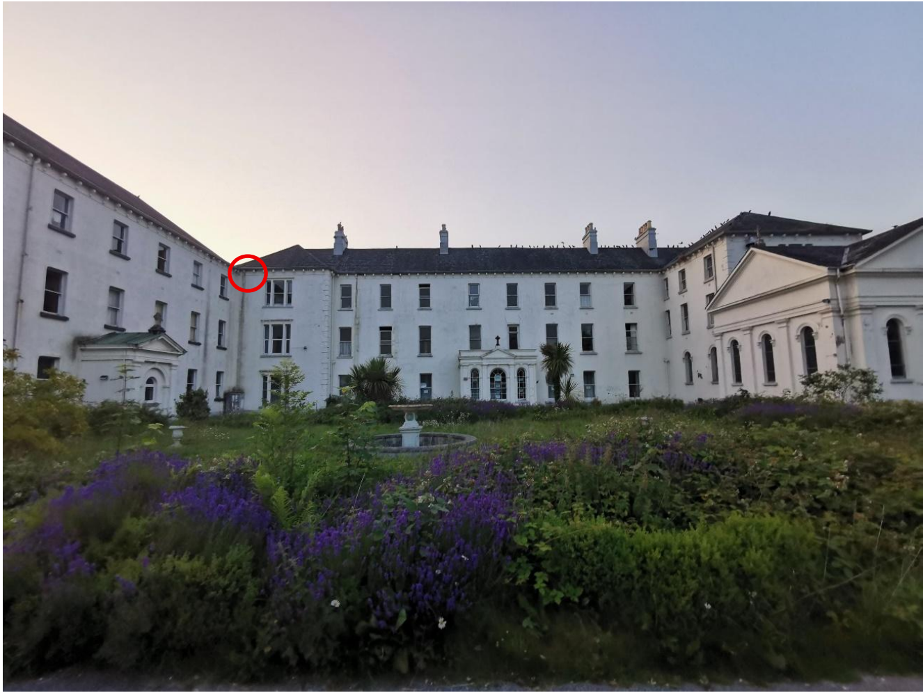
Figure 4-3: Emergence points for Soprano Pipistrelle from southern face of building (1 May 2025)
