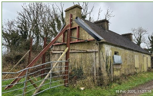
Plate 1 North and eastern aspects of existing Lesser Horseshoe Bat roost.
