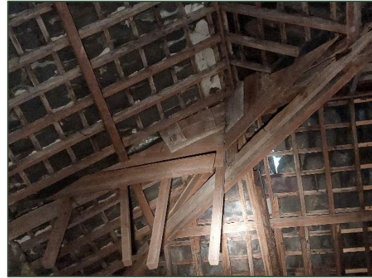
Plate 3.7 Example of complex joinery at hip-roof sections of Apartment 11.
