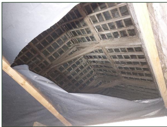
Plate 3.8 View of Apartment 10 attic.
