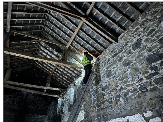
Plate 3.5 Surveyor at height inspecting stonework crevices and roof structure.
