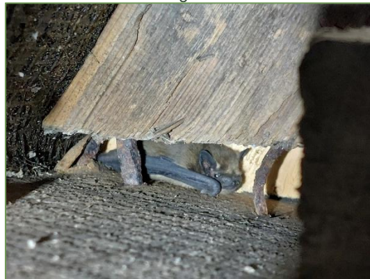
Plate 3.3 Common Pipistrelle roosting in the ridge beam joinery within the attic of Lissardagh House.
