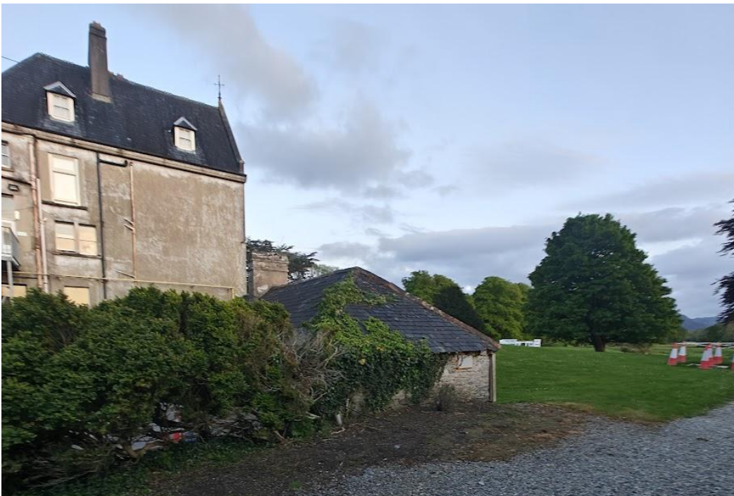
Plate 0-3: NW face of laundry room.
