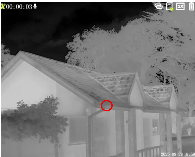
Plate 5-4: Cabin adjacent to Hotel (Cottage 2 Location)
