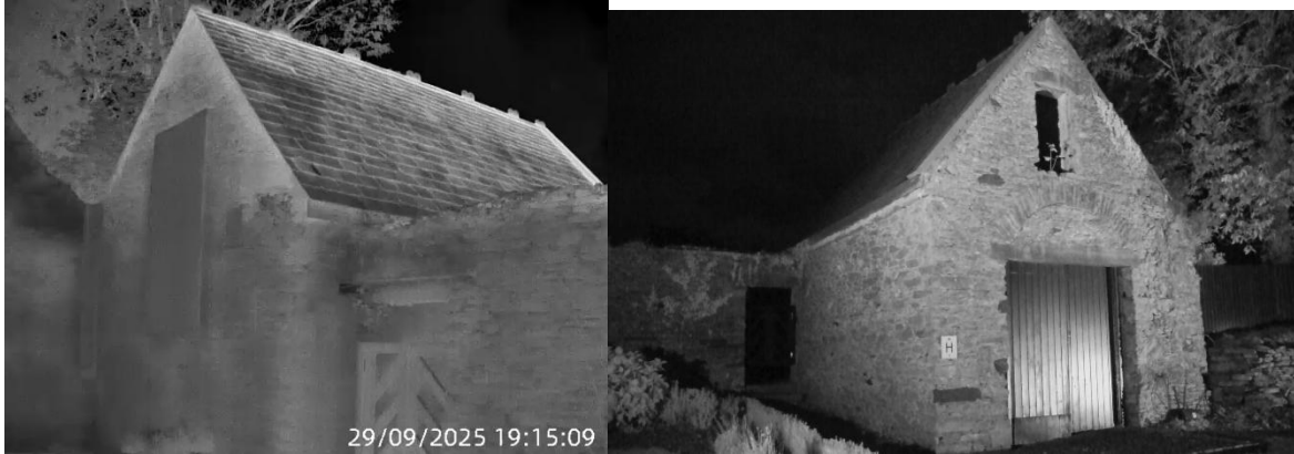
Plate 5-3: Storage Shed (Cottage 1 front)
