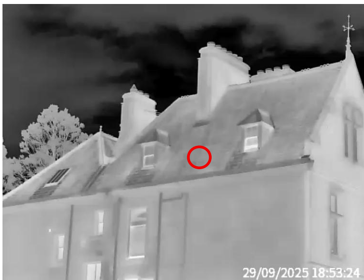
Plate 5-1: West side of Cahernane House Hotel
