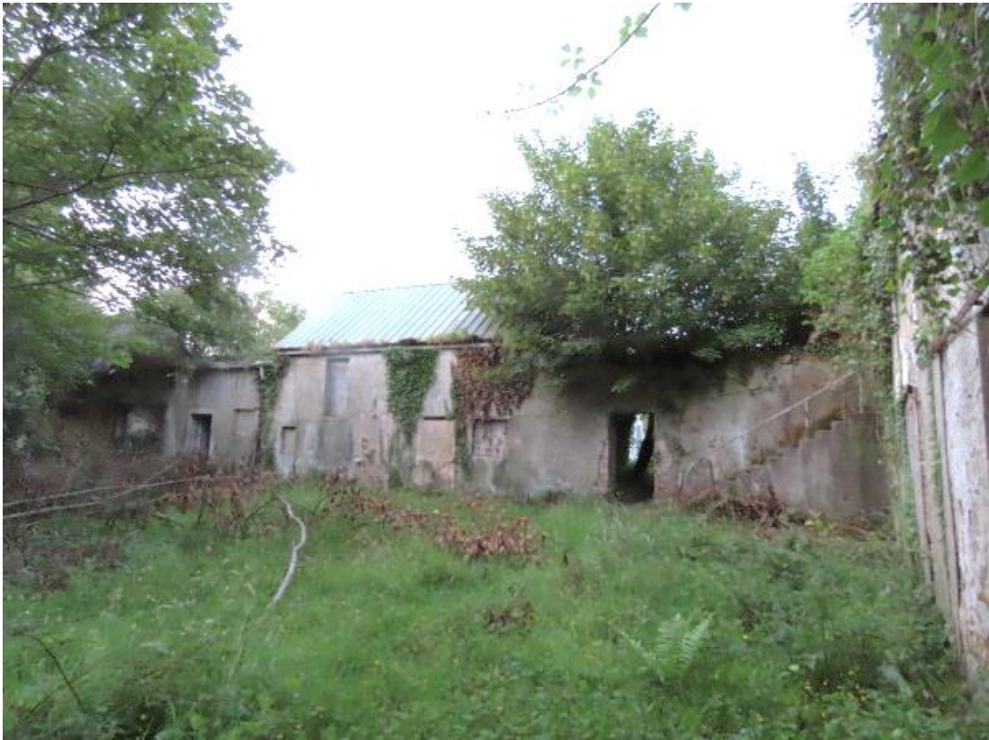
Figure 4. Exterior of outbuildings, showing the only structure with an intact roof
