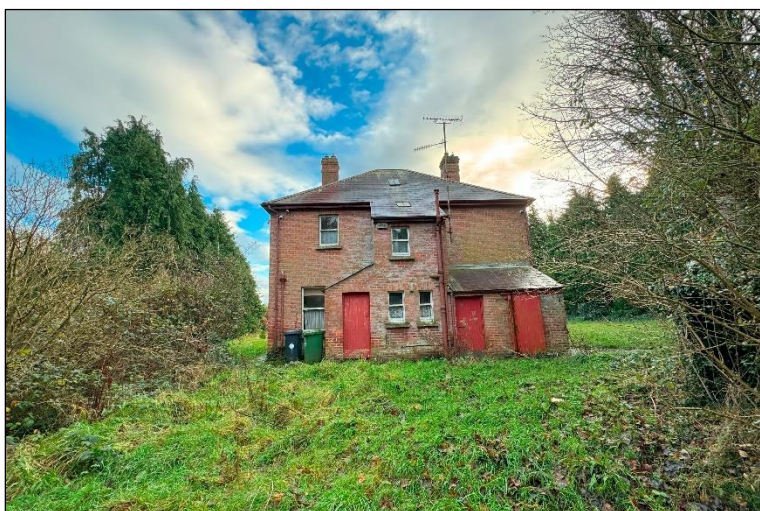
Plate 6 Rear view of the main building on the proposed development site (winter survey).
