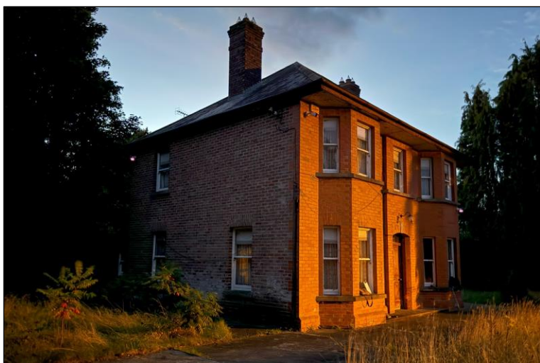
Plate 1 Existing main building (Highfield House) on the proposed development site.
