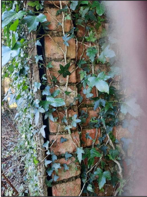
Plate 3-31 Old ruin with red brick and plaster that is separating from the brick leaving a large gap.
