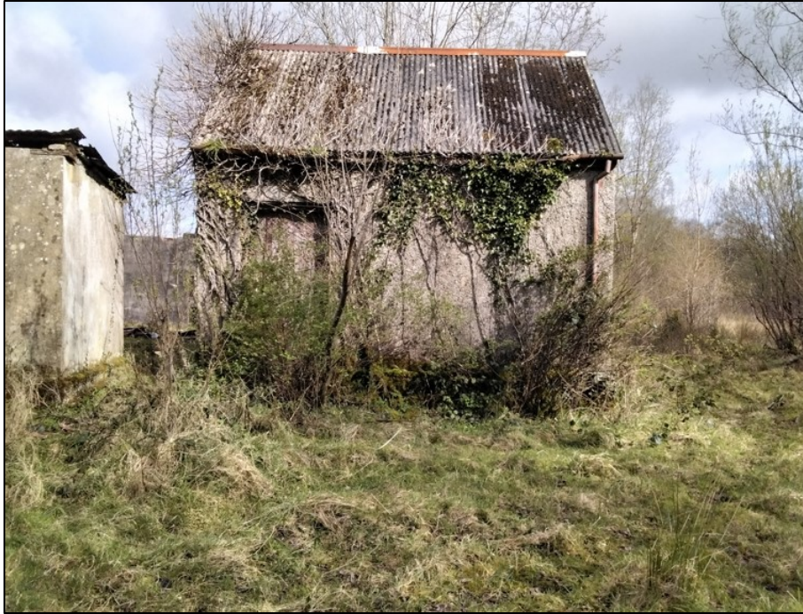
Plate 3-38 Shed adjacent to the derelict bungalow.
