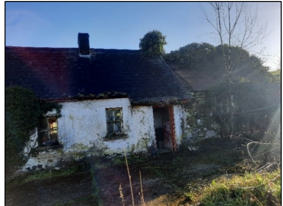
Plate 3-18 Southern Cottage B2 with cowshed attached to the north.
