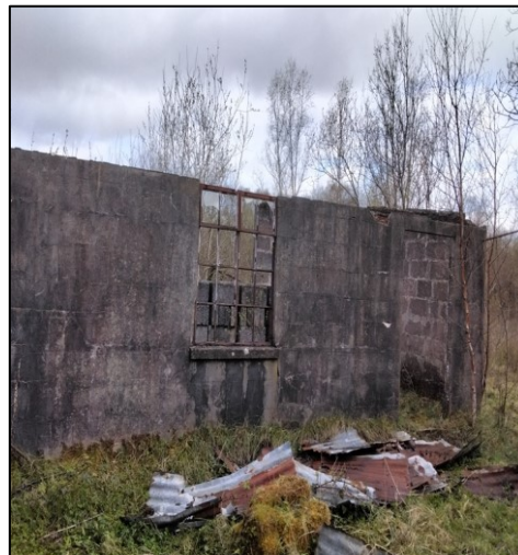
Plate 3-37 Extension to the rear of the derelict bungalow.
