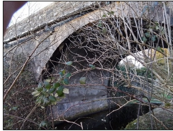
Plate 3-8 Southern aspect showing the plastered underside of the bridge.
