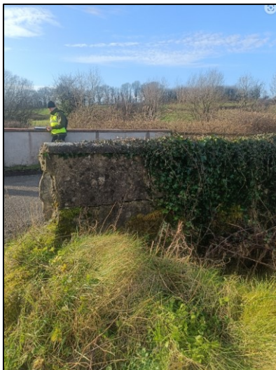
Plate 3-9 Bridge 3 Concrete pipe, with ivy cover and lime plaster over solid block bridge walls
