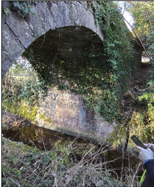
Plate 3-1 Arch bridge east side view.
