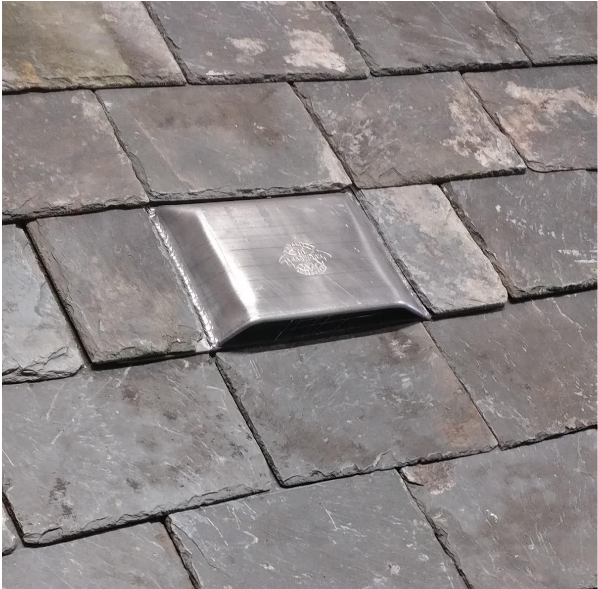
Photo 5: Bat access roost tile to be installed in the roof to provide access for common pipistrelle bats.
