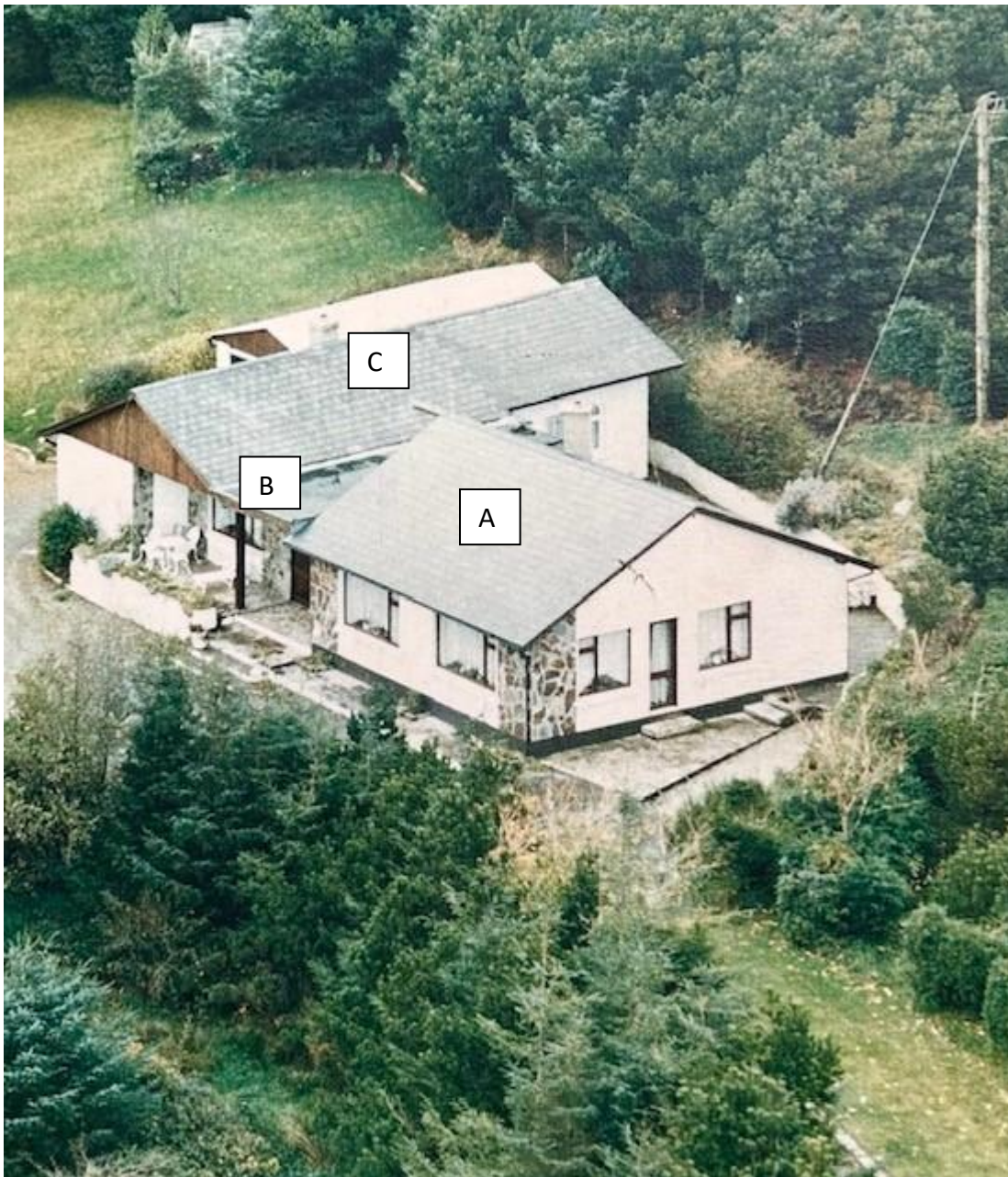
Photo 2: Aerial view of derelict bungalow, Coollick, Co. Kerry.
