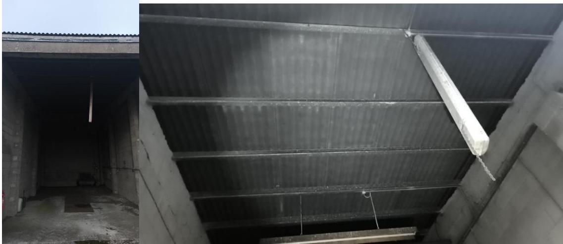
Asbestos roofed shed suitable for roosting.
