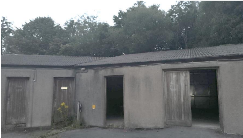
Asbestos roofed sheds suitable for bat roosting.
