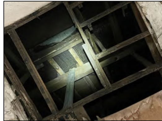
Plate 3-4 Cleeves factory attic space – roof lining
