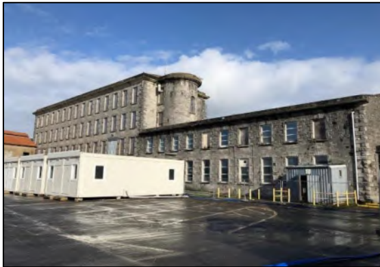
Plate 3-3 Cleeves Factory main building
