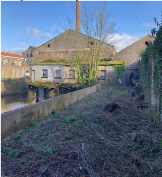
Plate 3-8 – Scrub WS1 to the west of the site & Office and cold store building, B14, to the right of the image, western elevation of workshop building, B13, in the background & a portion of the reservoir to the left of the image.
