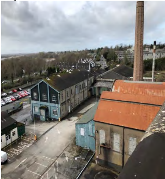
Plate 3-4 – Electrical station/ Storage Unit, B10, in the foreground & offices and workshop buildings, B15 & B13, in the background– facing southwest
