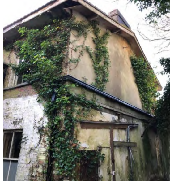
Plate 3-7 – Southern & eastern elevation of Unoccupied Dwelling, B1
