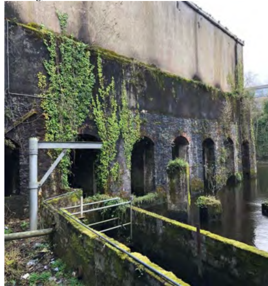
Plate 3-9 – Northern elevation of the Arch tunnel within the site
