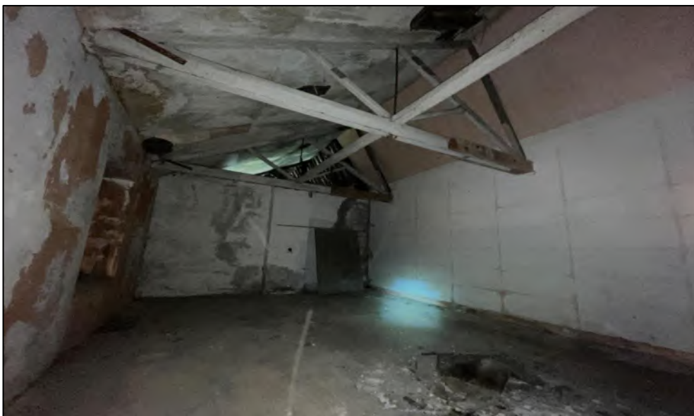
Plate 3-2 Interior of Building 14.
