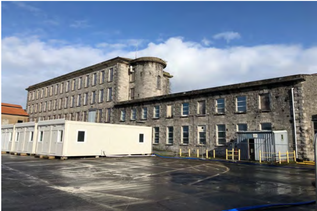
Plate 3-1 Southern Elevation of the Cleeves Factory within the site to the left of the image and Building B8 to the right of the image. Temporary HSE prefab units in the foreground of the image.
