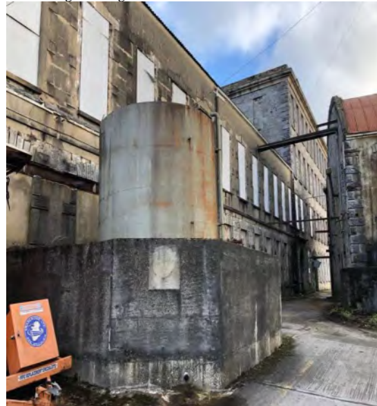
Plate 3-5 – Storage Unit, B11 to the left of the image– southern elevation
