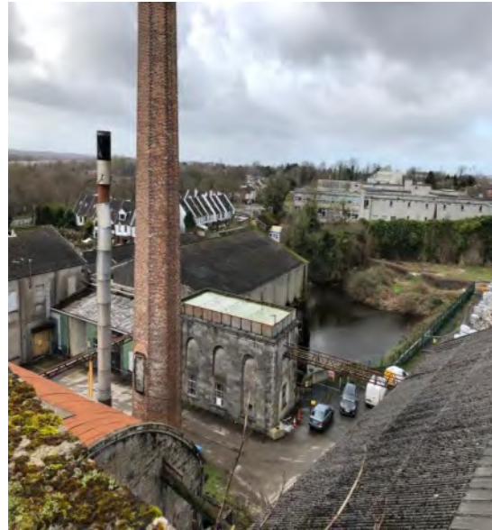
Plate 3-3 – Workshop, office and storage unit buildings, B13 & B14, to the left of the image and the reservoir to the right of the image– facing west
