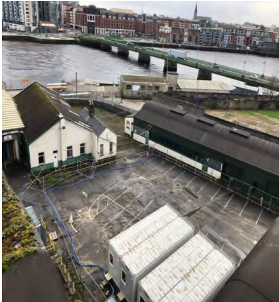
Plate 3-2 – Office buildings and storage units, B3 & B4, in the foreground & the rowing club building in the background– facing southeast
