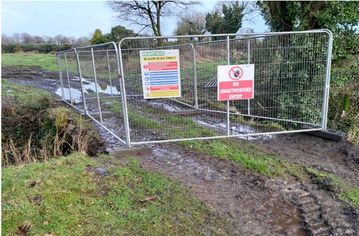
Figure 1: Current condition of B2346.
