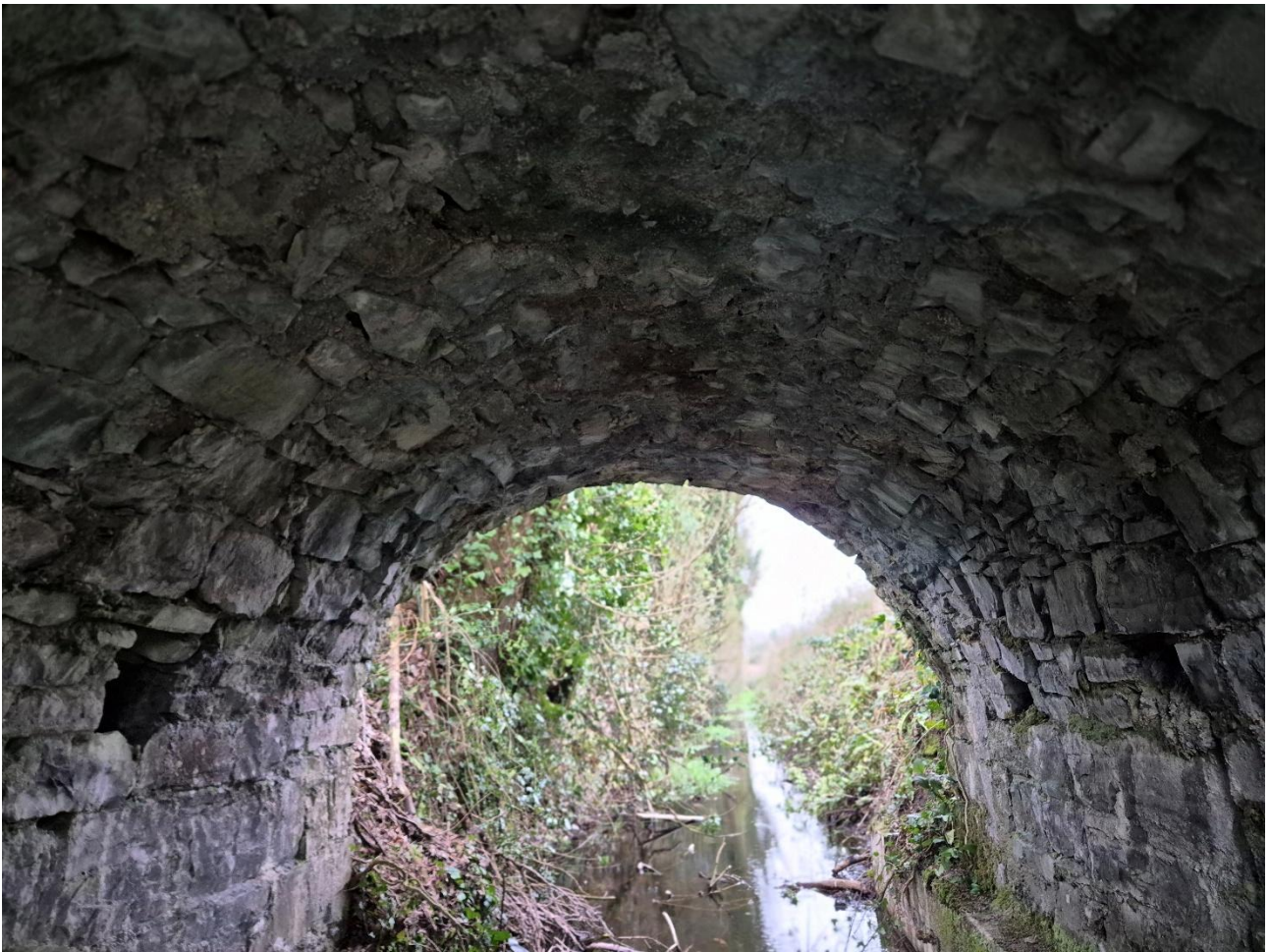
Plate 1d: Remainder view of in Drumcree Bridge, Co. Westmeath.
