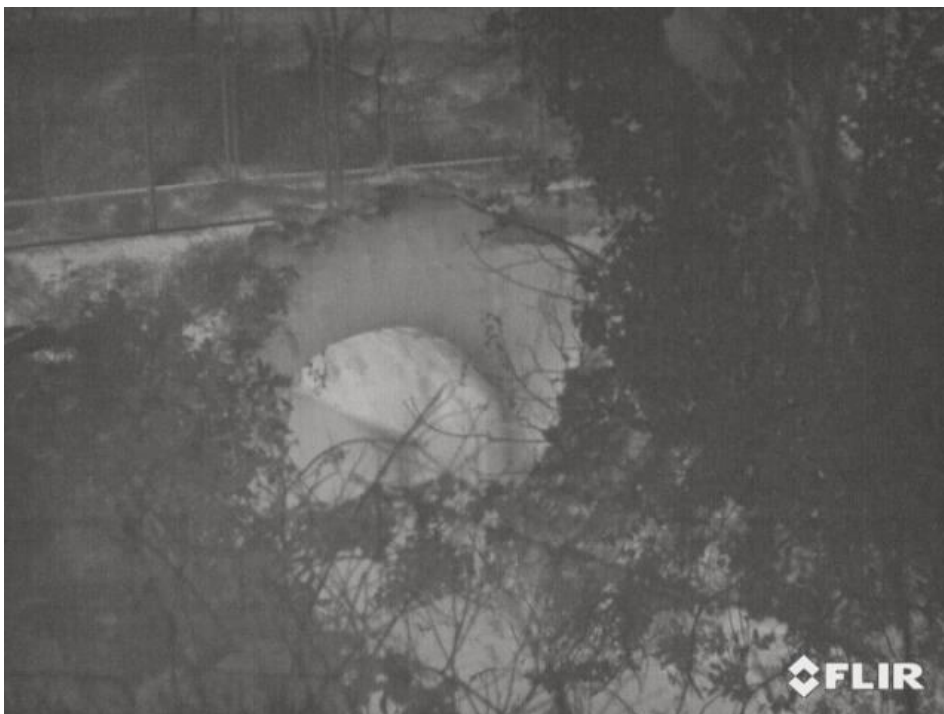
Figure 5b: Screenshot of thermal imagery footage recording of otherwise of Drumcree Bridge, Co. Westmeath.
