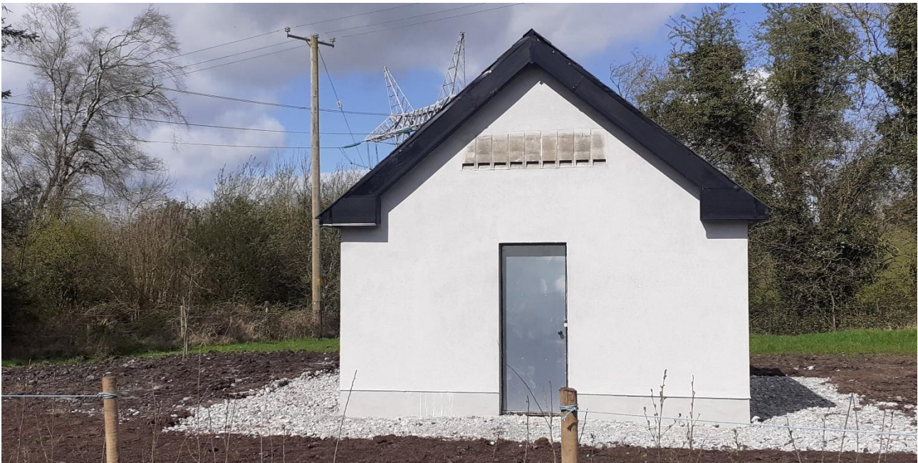
Plate A: Finished bat house with bat tubes (south facing external wall), Oldstreet Substation Bat House, Co. Galway.
