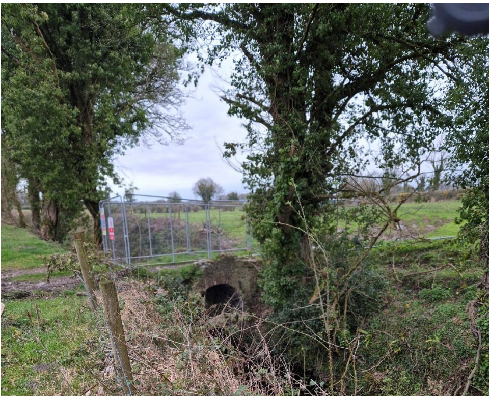
Plate 2: View of in Drumcree Bridge, Co. Westmeath.
