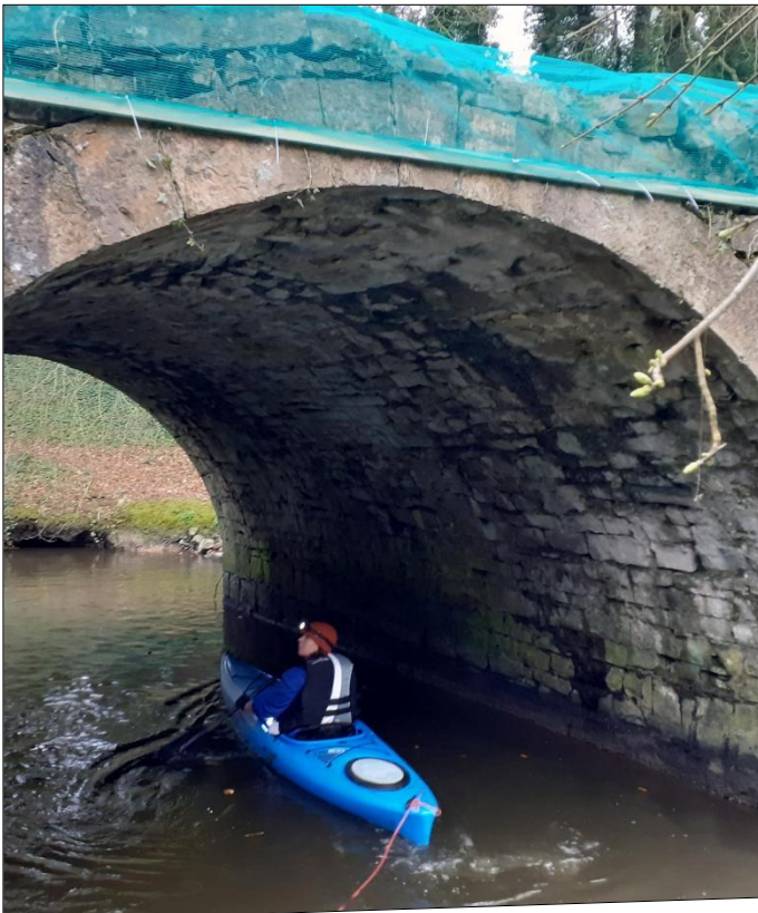
Plate 4: Claddy Bridge, Bective, Co. Meath – preparation work prior to works.
