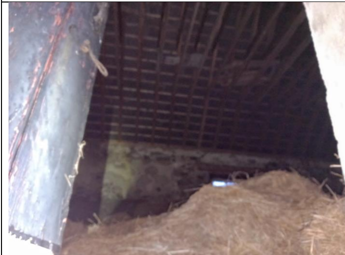
Interior of loft space Stable B
