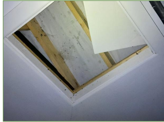
Plate 3.2 Attic hatch within pump room.
