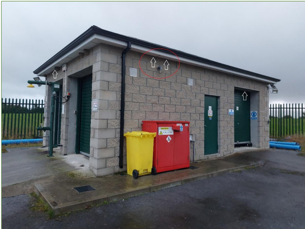
Plate 3.11 View of western side of Pump House building, arrows indicate observed access/egress points. Red circles indicate those observed to most commonly observed to be used.
