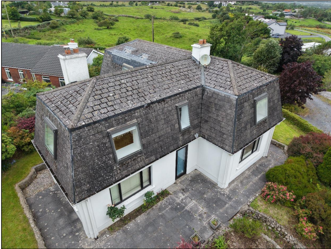
Figure 10. Mansard roof
