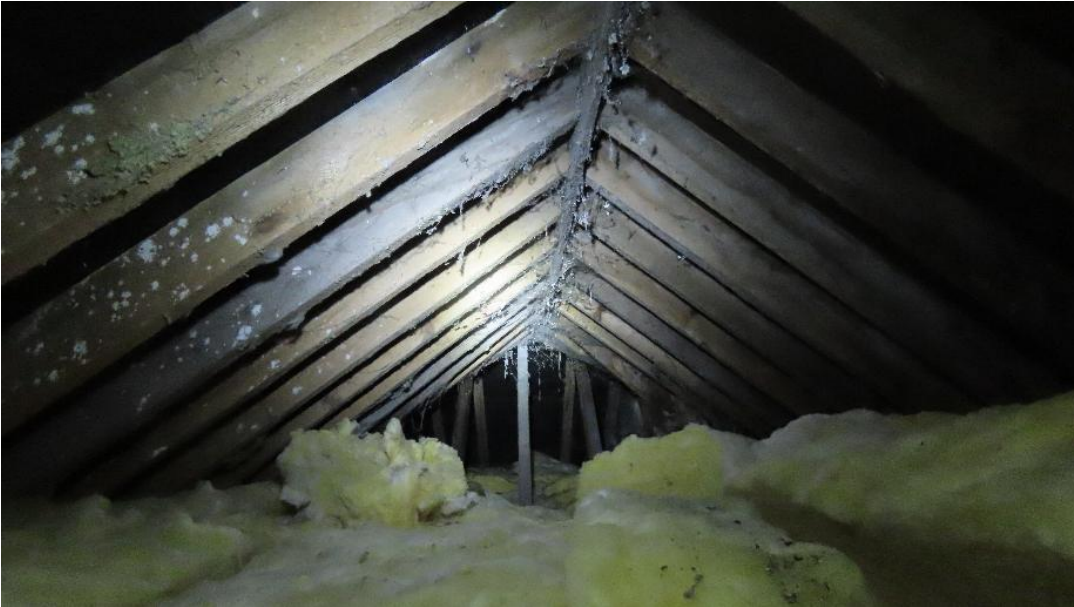
Photo 19 – view of attic space of dwelling house
