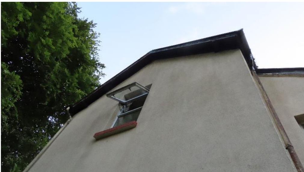
Photo 2 – open upstairs window on eastern gable through which two Brown long-eared bats emerged from the house
