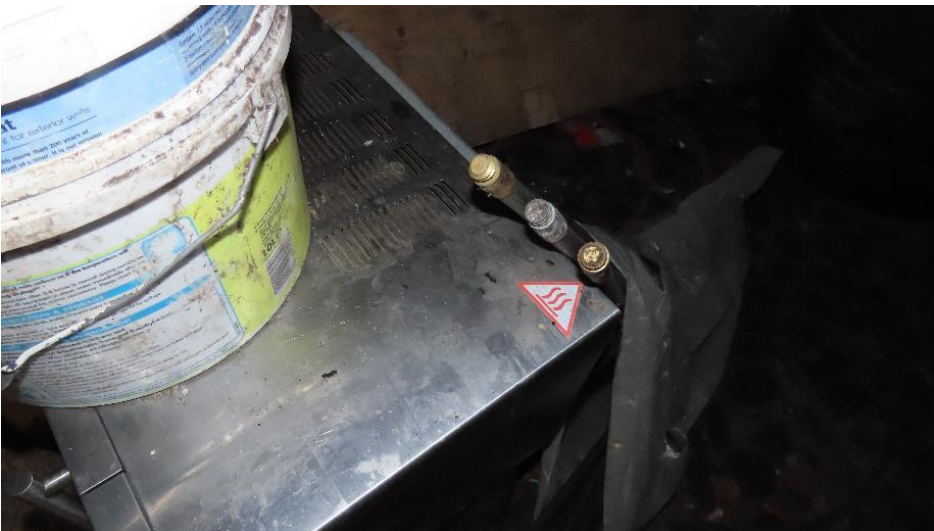
Photo 31 – some scattered bat droppings of Brown long-eared bat in lower building
