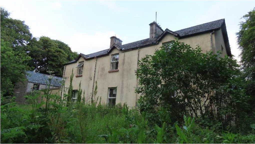
Photo 4 – western elevation of dwelling house
