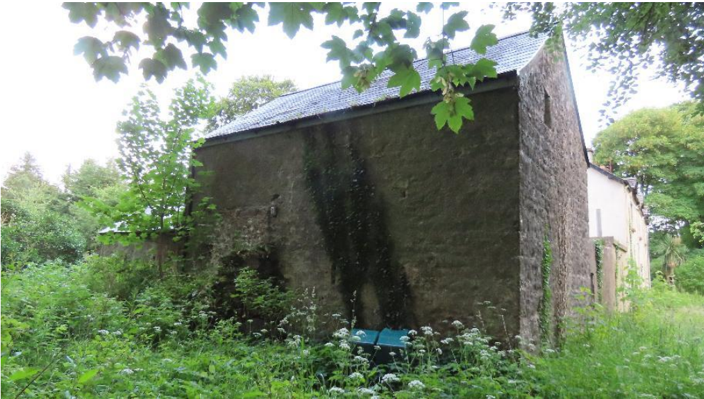
Photo 27 – rear elevation and western gable of granary
