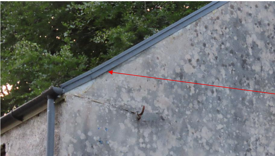
Photo 23 – close up of exit point on eastern gable of granary building
