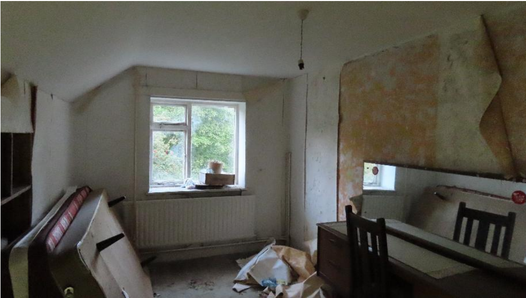
Photo 10 – bedroom upstairs in dwelling house
