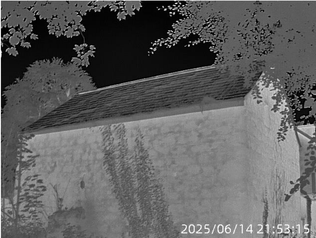
Photo 34 – Thermal photo of rear and western elevation of granary
