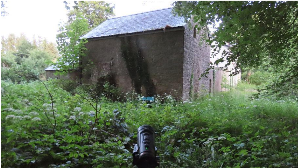
Photo 28 – thermal camera trained on rear and western gable of granary
