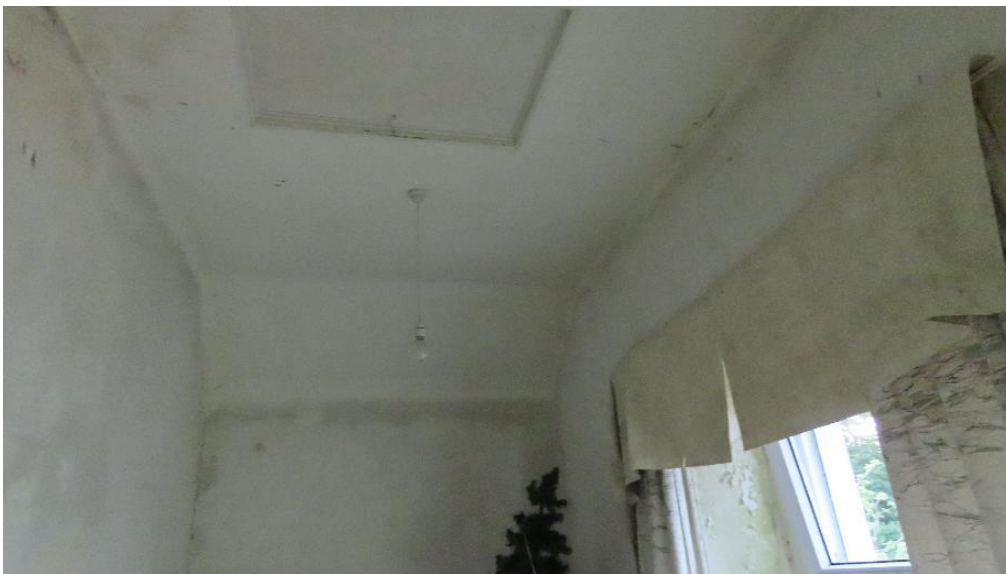
Photo 9 – trap door to attic space
