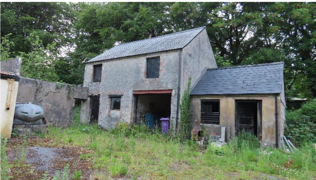
Photo 21 – front elevation of granary. Swallows nesting in lower building
