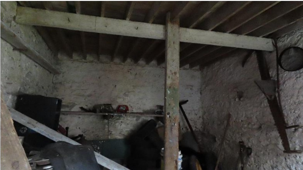
Photo 25 - ground floor of granary building used for storage. Wooden loft floor above
