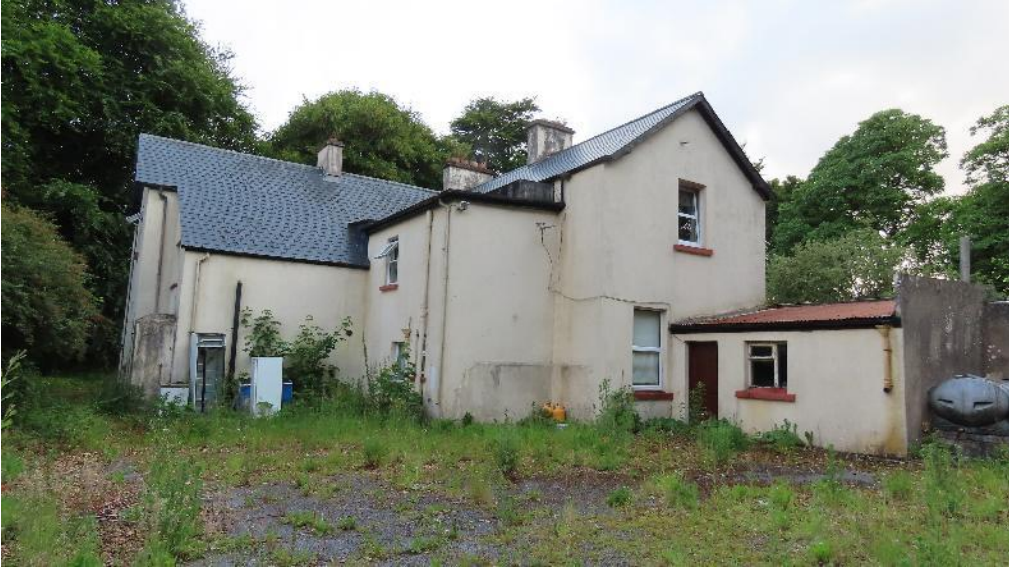
Photo 3 – rear elevation of dwelling house
