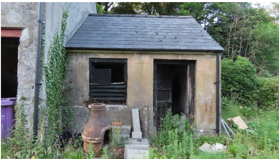
Photo 29 – lower building attached to granary with swallows' nests on roof timbers
