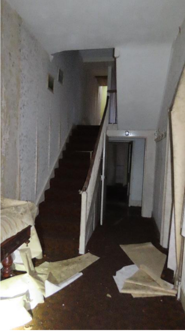
Photo 5 – stairs in dwelling house
