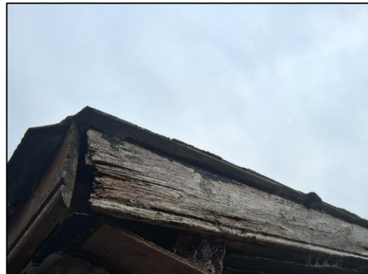
Plate 4-6 Broken barge board on the shed to the north of the main building
