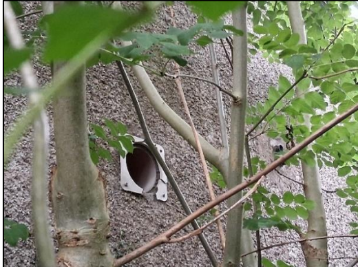
Plate 4-3 Air vent to the northeast of the main school building
