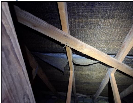
Plate 4-7 Underlay in the attic under tiled roof
