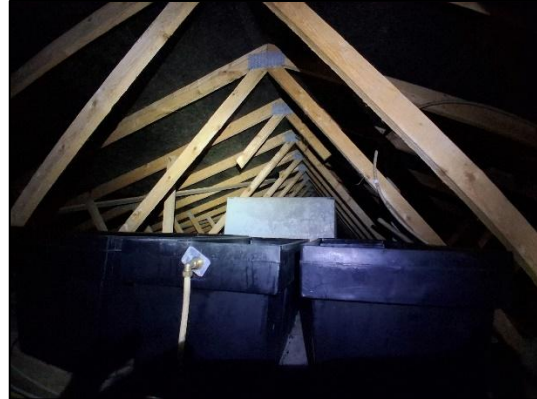
Plate 4-10 Attic of the Art Building
