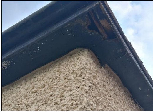
Plate 4-1 Soffit of the most eastern building
