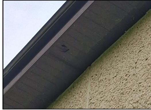
Plate 4-2 Soffit to the south of the sport hall
