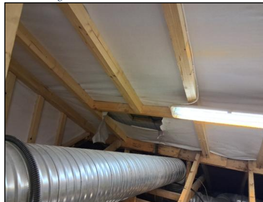
Plate 4-8 Insulation between the corrugated iron sheets of the recently renovated attic
