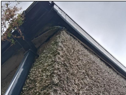
Plate 4-5 Gap between barge board and wall of the main building
