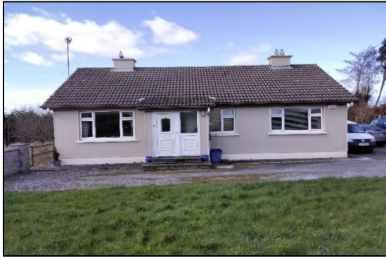
Plate 5-7 Bungalow for demolition with single attic space and two chimneys.
