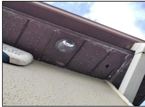
Plate 5-8 Southern aspect soffit with one hole.
