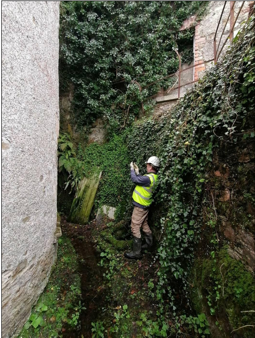
Photo 7. Fern and moss rich walls of the basement passageway.
