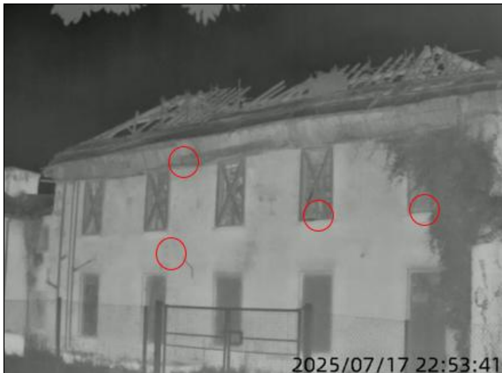
Figure 29. Emergence locations at the rear of the house - recorded by NVA 3.
