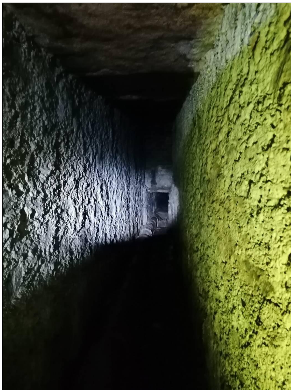
Photo 13. The tunnel in front of Kilmacurragh House.
