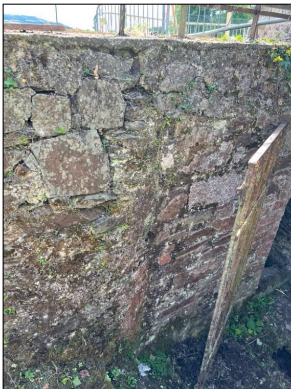
Photo 10. Bryophytes on mortar in basement wall to NE of house (at bottom of steps).
