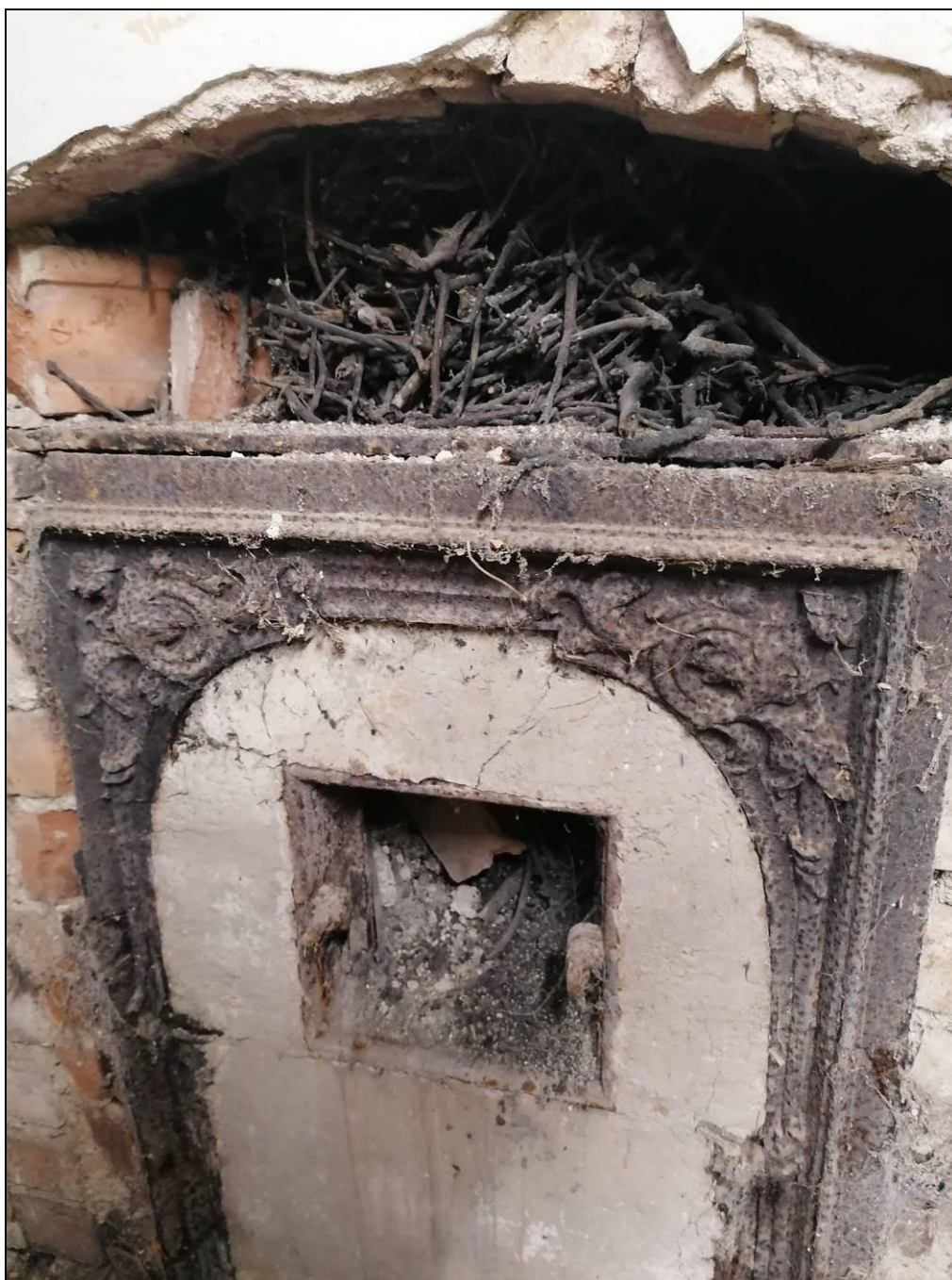
Photo 30. Jackdaw nest in fireplace/chimney.
