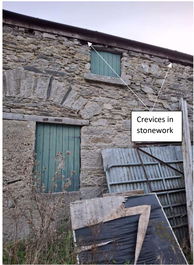
Plate 2. Outbuilding along the southwestern boundary
