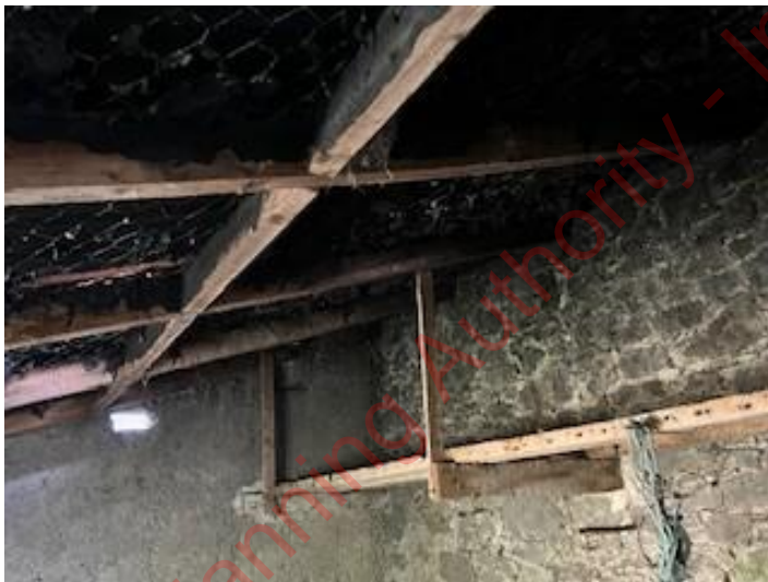
Example of S4's internals.
