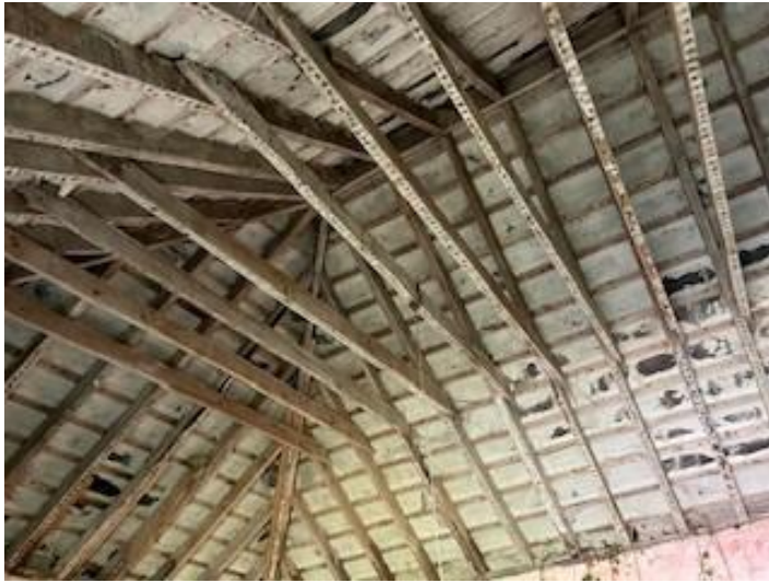
Example of B4's internal roof structure.
