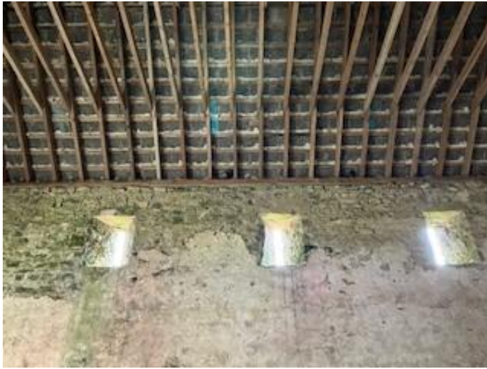
Example of B6's internal roof structure.
