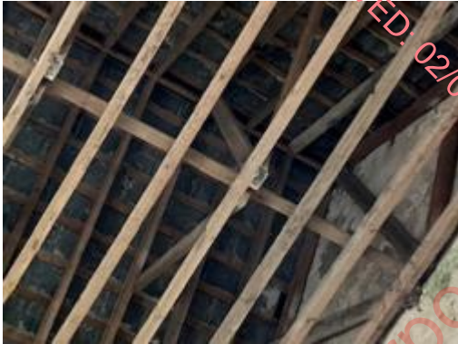
Figure xxiv: Roosting potential along central roof ridge beam.
