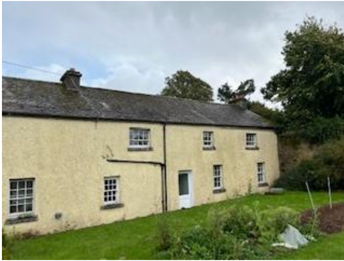
Western facing aspect of B5.
