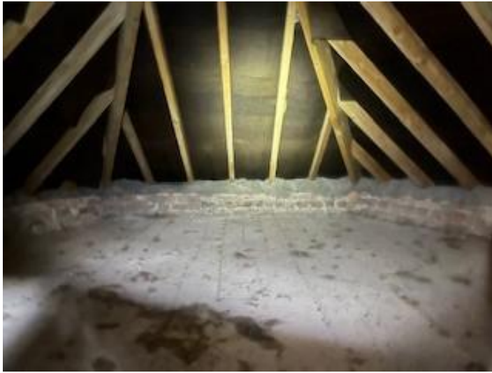
Example of loft space inside B1.
