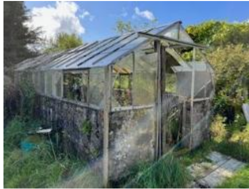
Figure 14: Northern and eastern facing aspects of B12.
