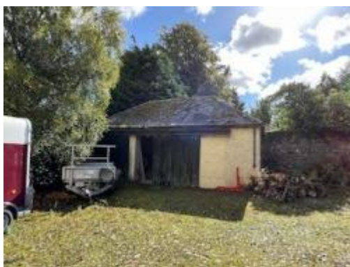
Figure 6: North facing aspect of B4.
