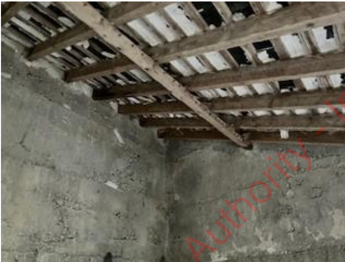
Example of B3's internal roof structure
