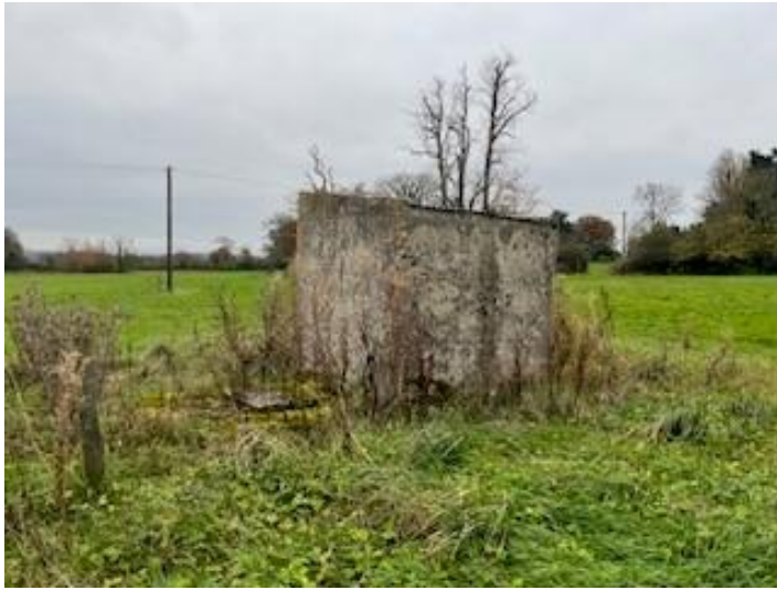
Eastern and northern facing aspects of S2.
