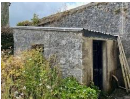
Figure 17: Eastern and southern facing aspects of S1.
