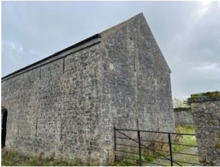
Northern and western facing aspects of B6.
