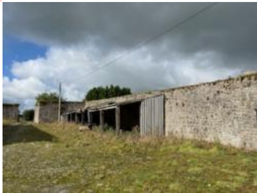
Figure 9: Eastern and southern facing aspects of B7.
