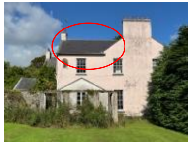
Figure x: southwestern gable with tight fitting newer slate roof tile.
