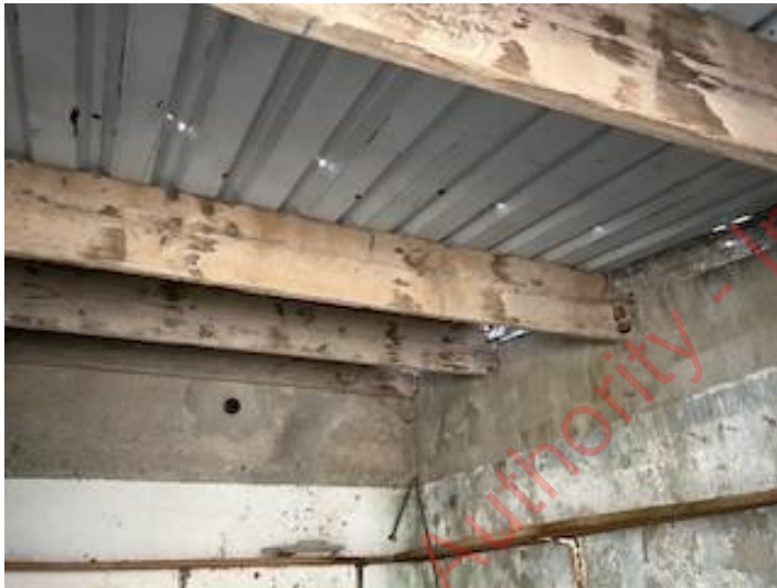
Example of S1's internals.
