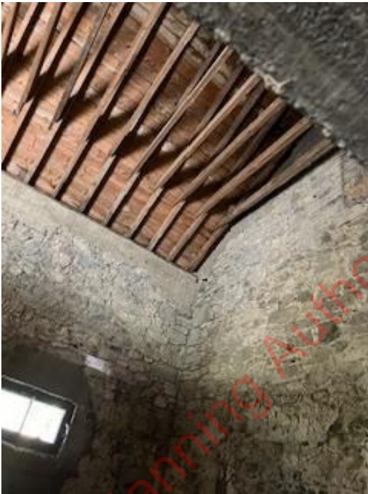
Example of internal roof structure within the stables section of B5.
