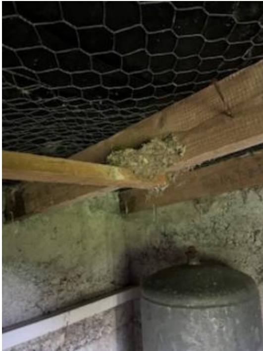
Example of S2's internals.
