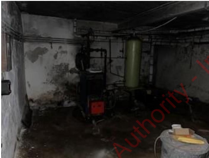
Example of underground cellar in B1.
