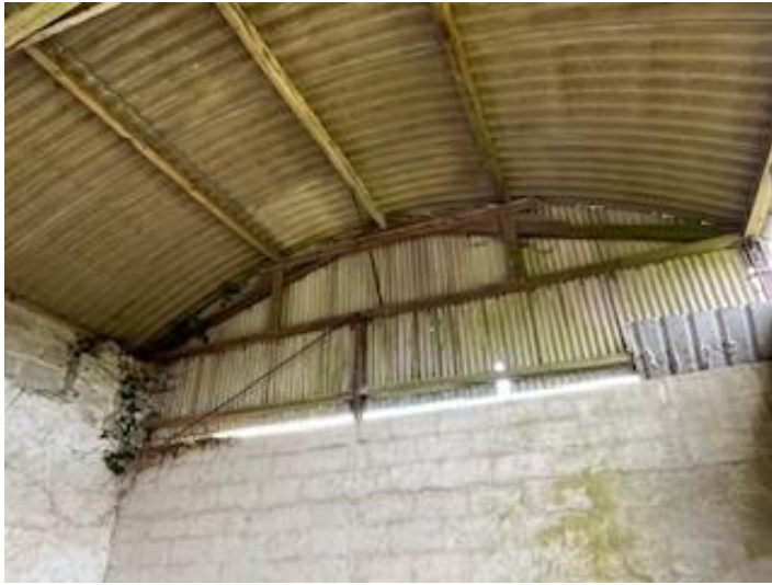
Example of B8's internal roof structure.
