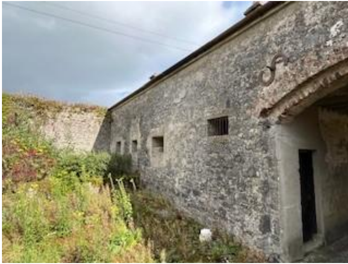
Western facing aspect of B5.
