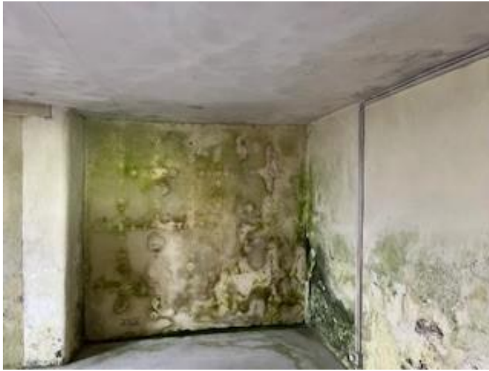
Example of underground cellar in B1.
