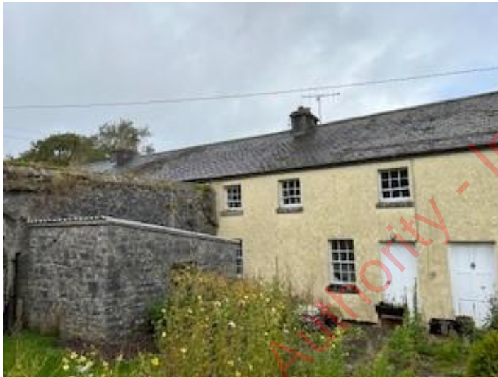
Western facing aspect of B5.
