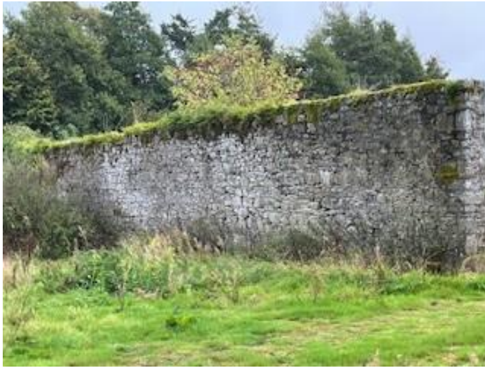
Example of walls found on site (S5).
