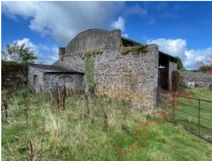
Southern and eastern facing aspect of B8.
