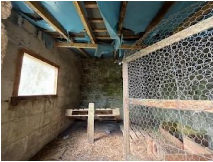
Example internal roof structure of lean-to section of B8.
