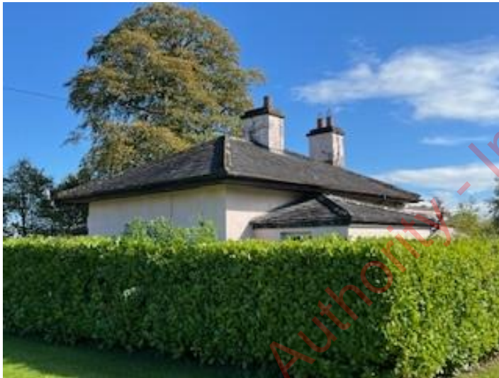
Northern and western facing aspects of B14.
