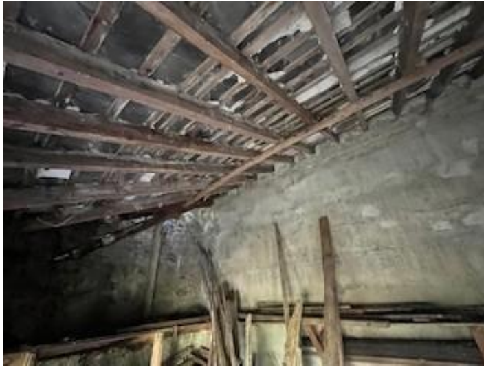
Example of B3's internal roof structure.
