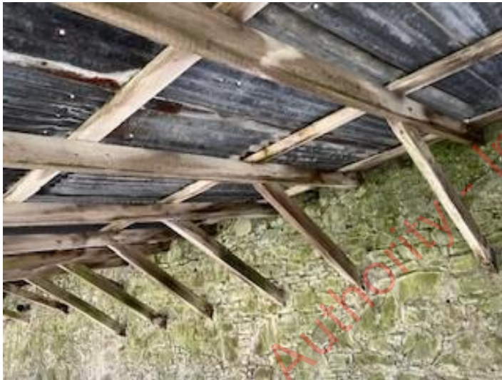
Example of B7's internal roof structure.
