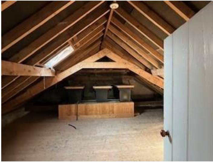
Example of loft space inside B1.
