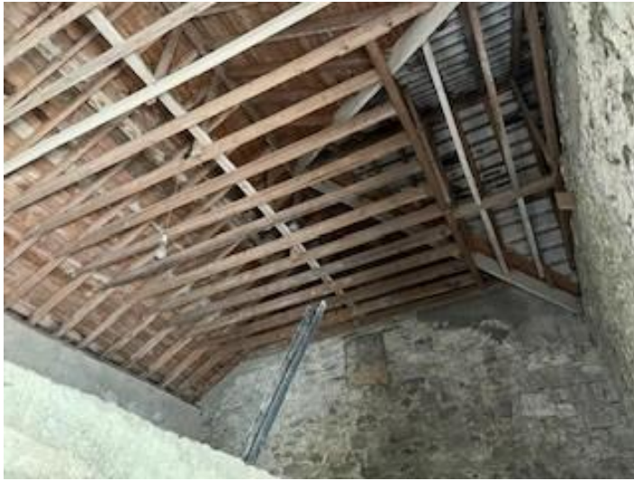
Example of internal roof structure within the stables section of B5.
