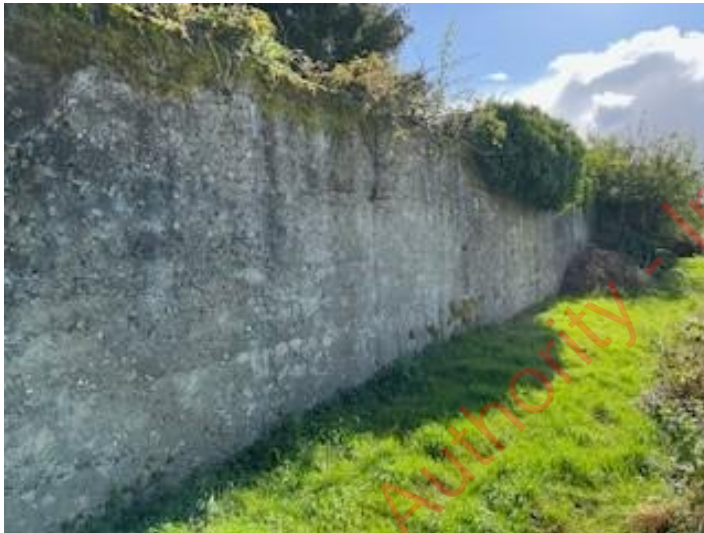
Example of walls found on site (S5).
