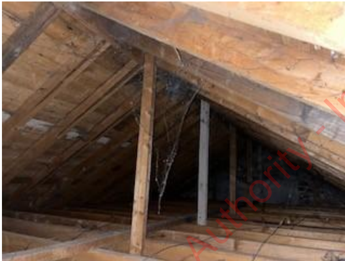
Example of loft space within the cottage section of B5.
