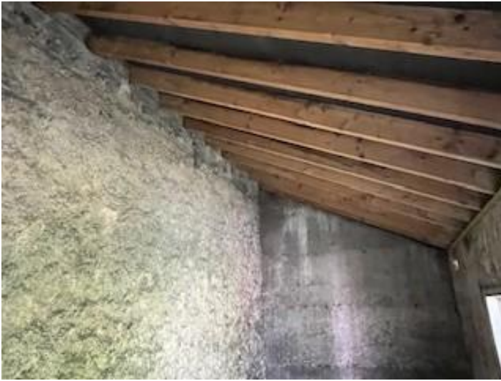
Example of B2's internal roof structure.
