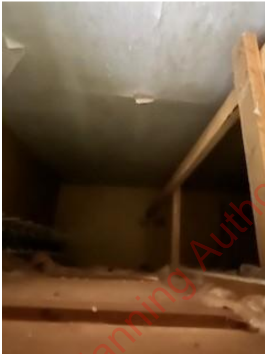
Example of B14's loft space.
