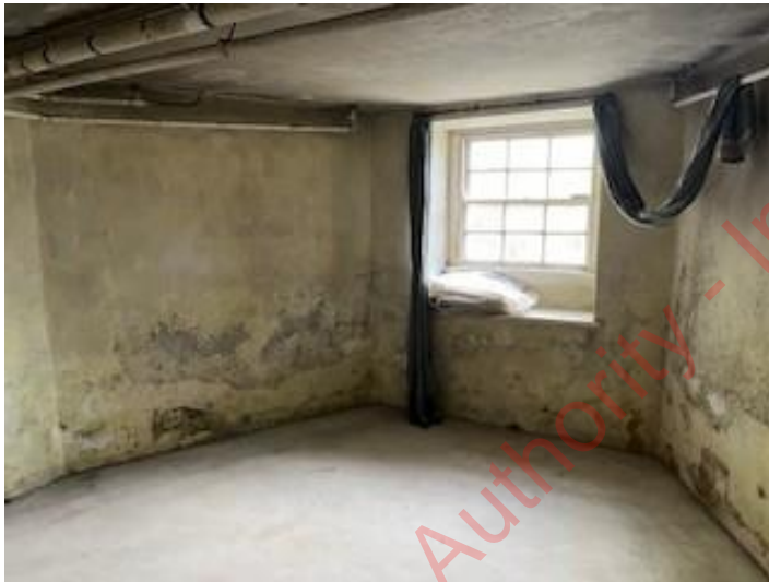
Example of underground cellar in B1.
