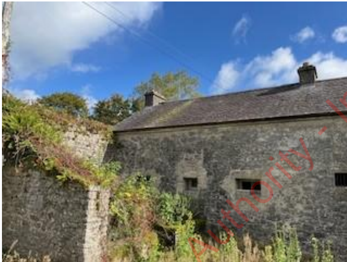
Western facing aspect of B5.
