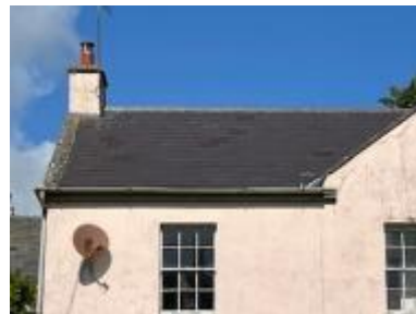
Figure x: southwestern gable with tight fitting newer slate roof tile.
