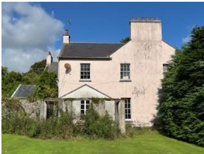
South facing aspect of B1.
