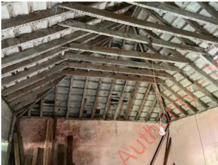
Example of B4's internal roof structure.
