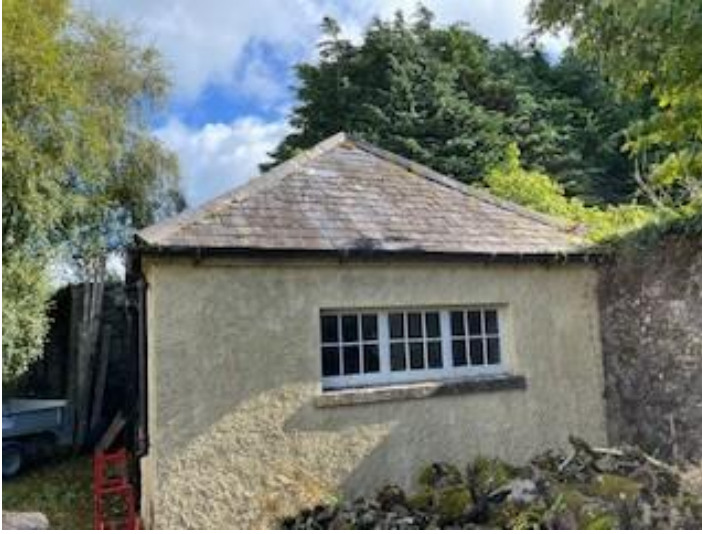
Western facing aspect of B4.
