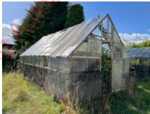
Figure 13: Northern and eastern facing aspects of B11.
