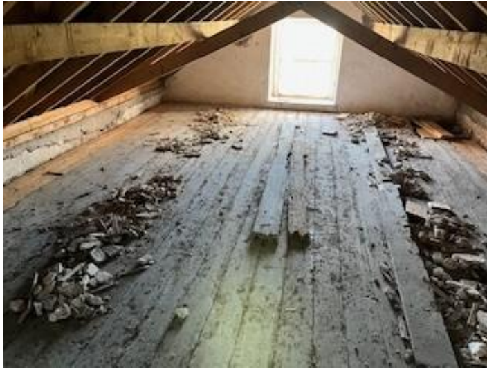
Example of loft space inside B1.
