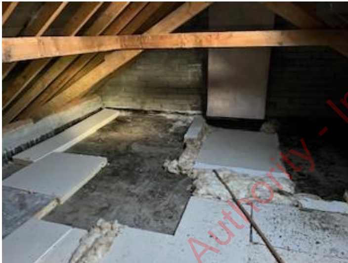
Example of loft space inside B1.
