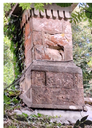
Existing Chimney to Gate lodge
