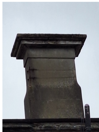
Existing rendered chimney
