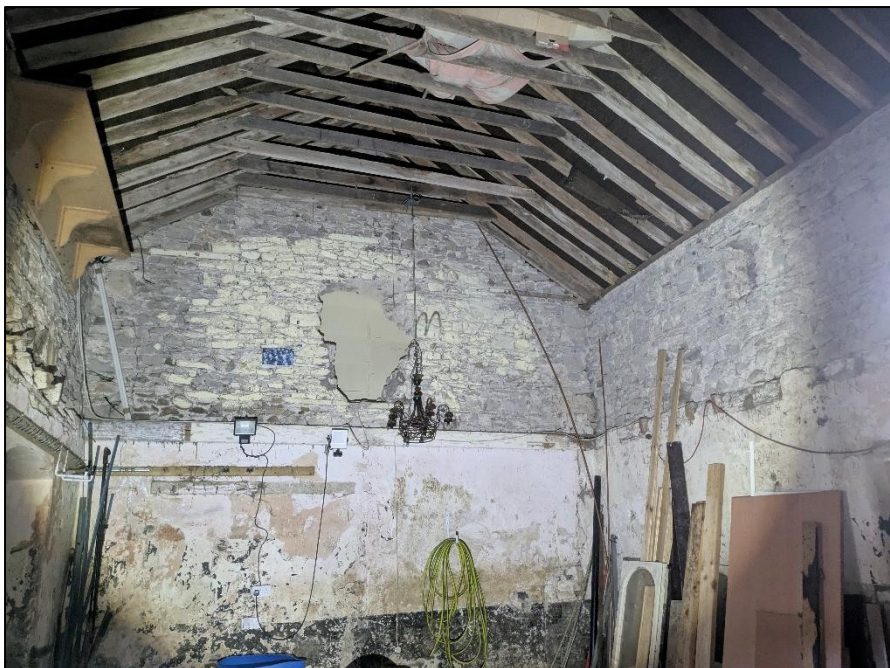
Plate 3-5. Northern-most section of subject building
