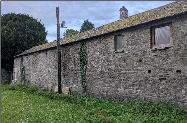
Plate 3-2. Rear of subject building.
