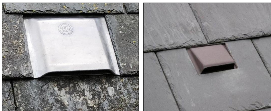
Plate 4-1. Example bat access tiles / vents ( 'Just Lead' , 'Beddoes' ).
