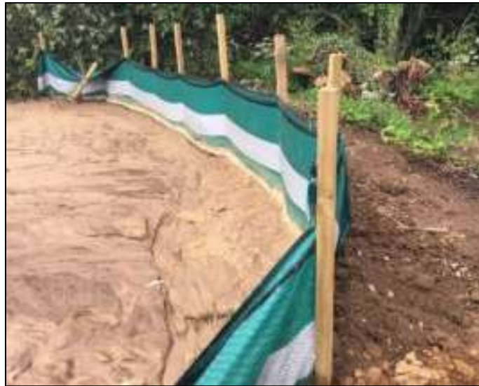
Figure 2-3 Typical Silt Fence
