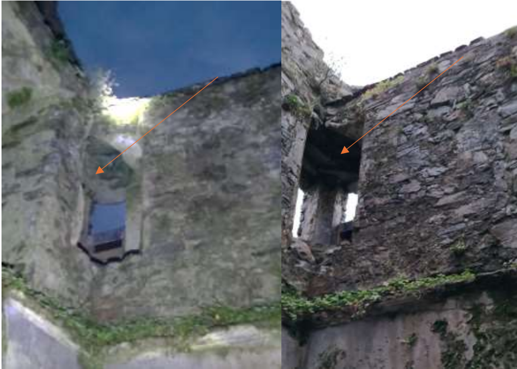
Red arrow – Main roost area within building
