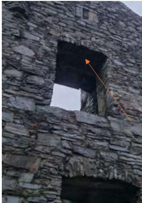
Soprano pipistrelle roost in stonework
